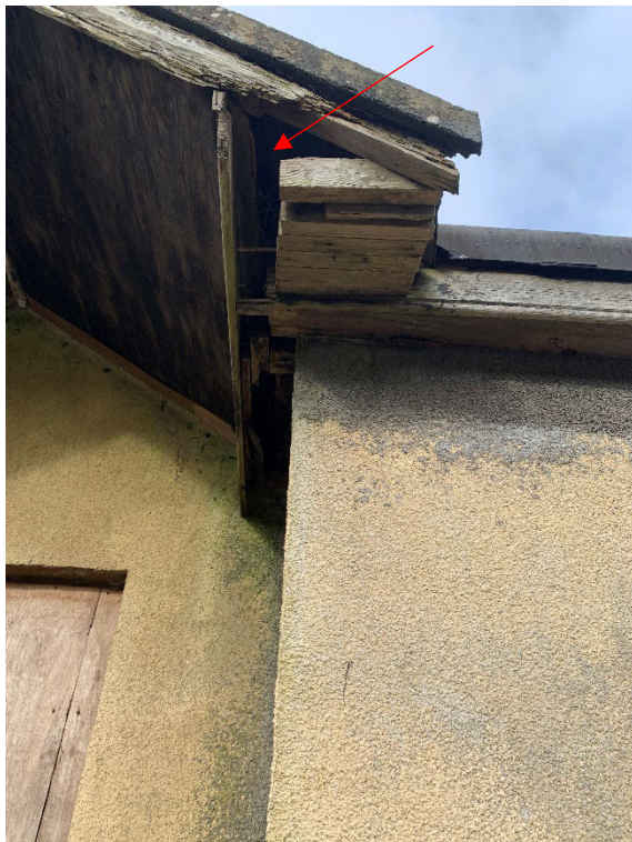
Plate 3-2: Suitable entry/exit point via gaps in soffits
