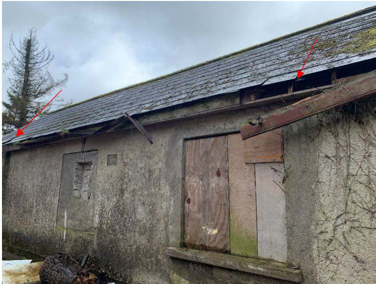
Plate 3-3: Holes in soffits and raised and slipped tiles
