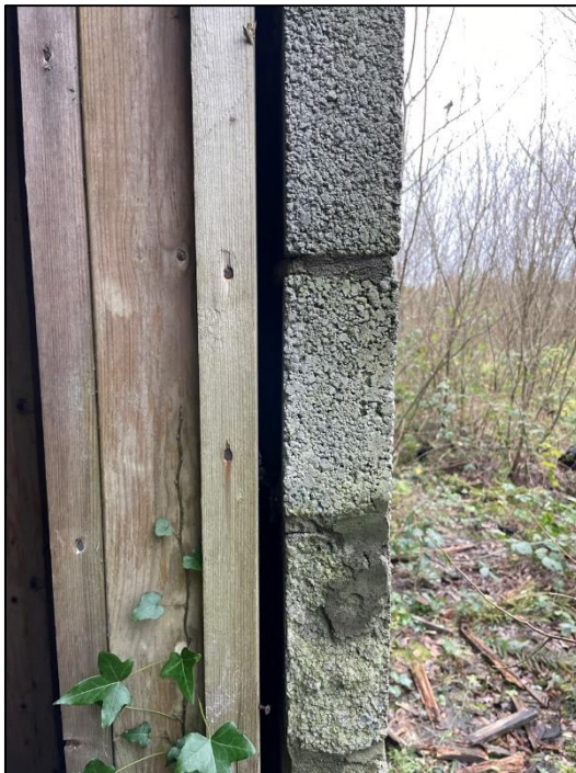
Plate 4-5 Two centimetres gap between timber cladding and exterior brick wall in houses 1 to 7
