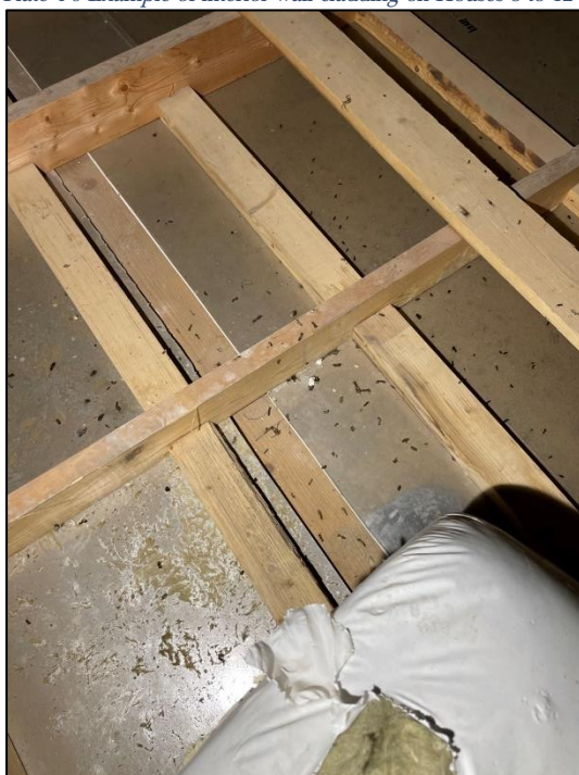
Plate 4-7 Bat droppings accumulation found on House 10 attic
