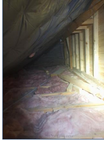
Plate 4-4 Attic with underfelt lining and loft insulation
