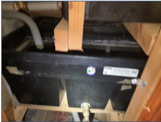
Plate 4-5 Uncovered water tank within the attic
