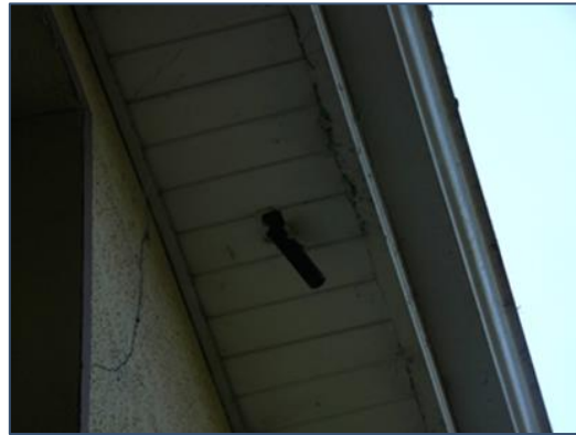
Plate 4-6 Possible bat access point at the soffit, next to a pipe
