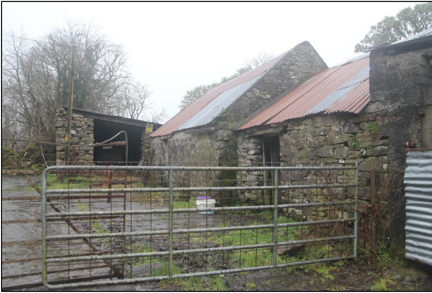
Plate 4 Site with existing sheds with hardstanding. All with Bat Roost Potential.
