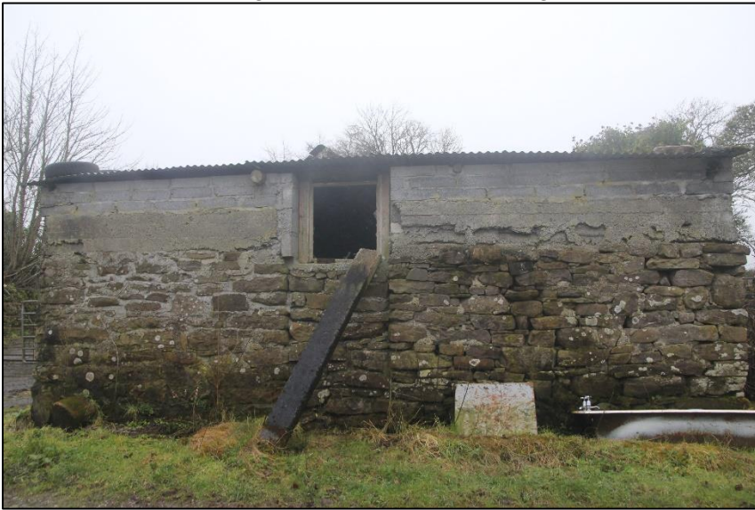
Plate 2 Site with existing sheds with hardstanding. All with Bat Roost Potential.
