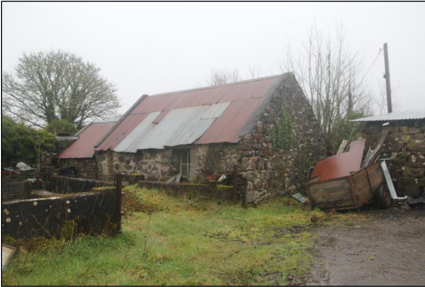
Plate 1 Site with existing sheds with hardstanding. All with Bat Roost Potential.
