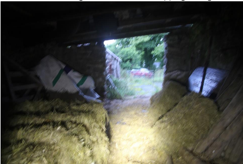
Plate 22 Building 1 Interior with bat droppings – August 2024
