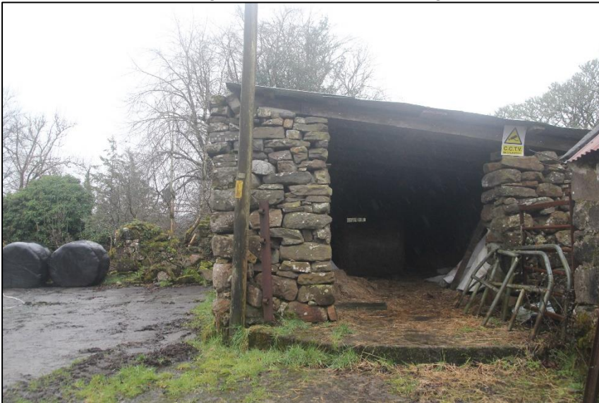
Plate 3 Site with existing sheds with hardstanding. All with Bat Roost Potential.
