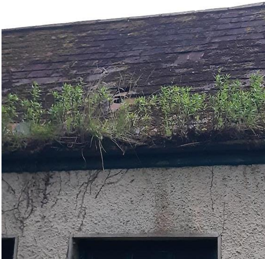
Plate 2. Hole in roof of stable block.
