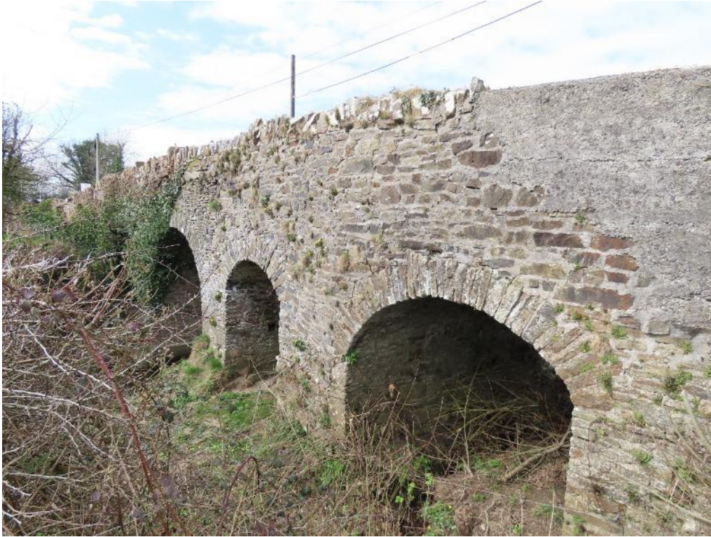
Boleybeg Bridge North
