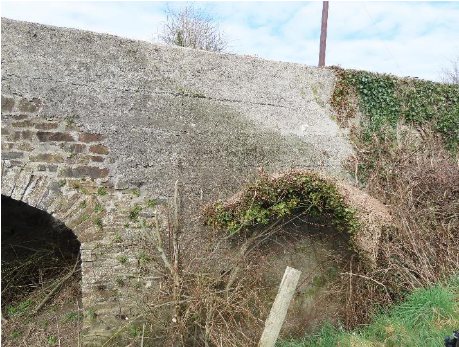
Photo 5 - section of parapet wall replaced with concrete blocks on eastern downstream side of bridge
