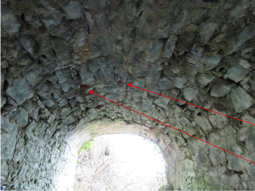
Photo 28 – two crevices marked for retention for bats under the arch
