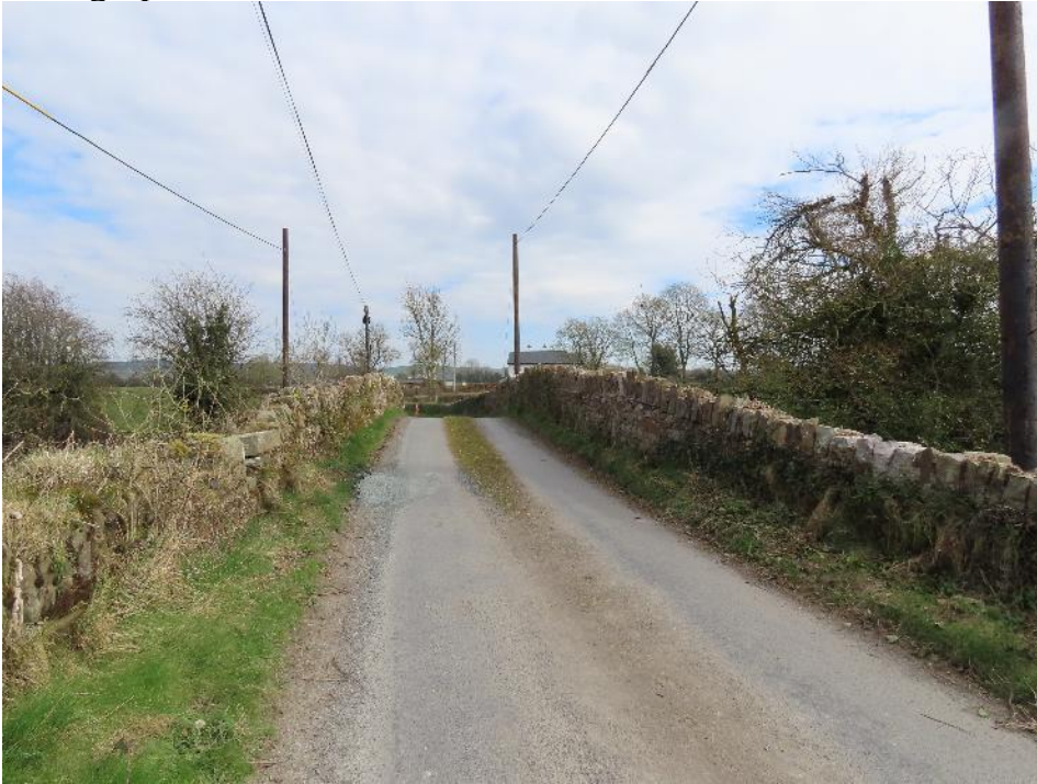
Photo 1 – looking east across Boleybeg Bridge North
