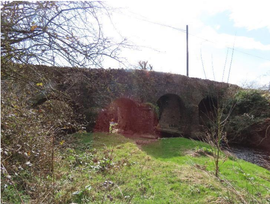
Photo 8 – upstream elevation of bridge from eastern river bank
