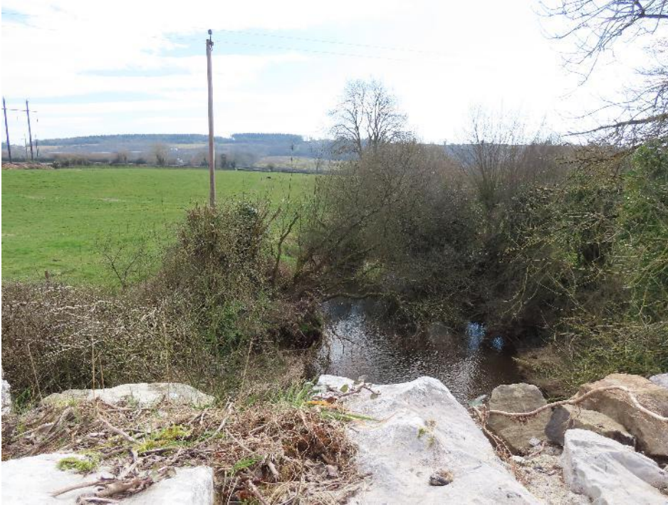
Photo 3 – Owenbeg River downstream of Bolybeg Bridge North
