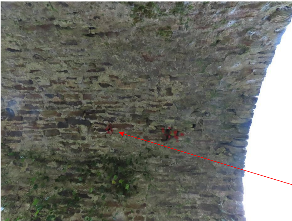
Photo 15 – three crevices marked for retention under Arch. A single Daubenton's bat was recorded in the crevice indicated approx. mid way under arch
