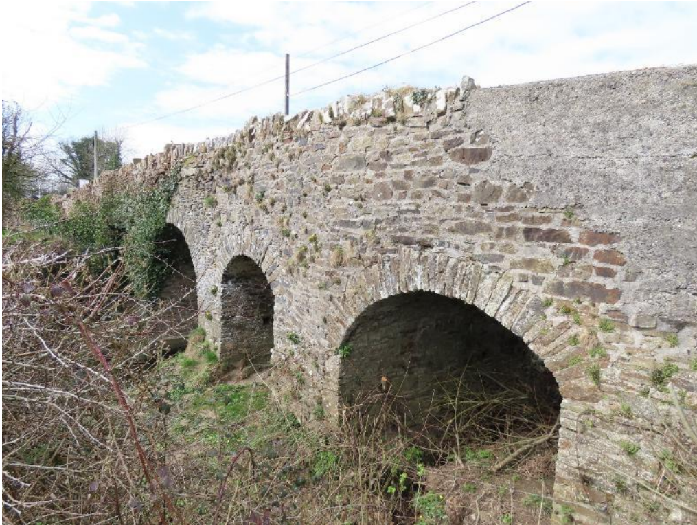
Boleybeg Bridge North
