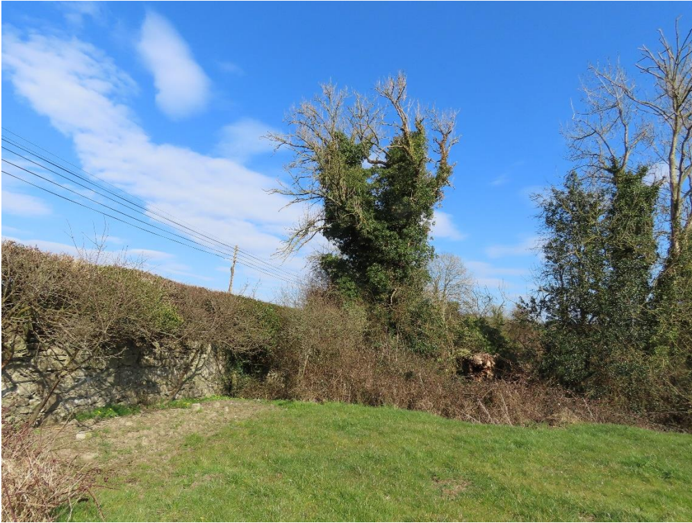
Photo 18 – mature ash tree with severe ash die-back growing very close to downstream side of bridge. A second mature ash has fallen beside this tree
