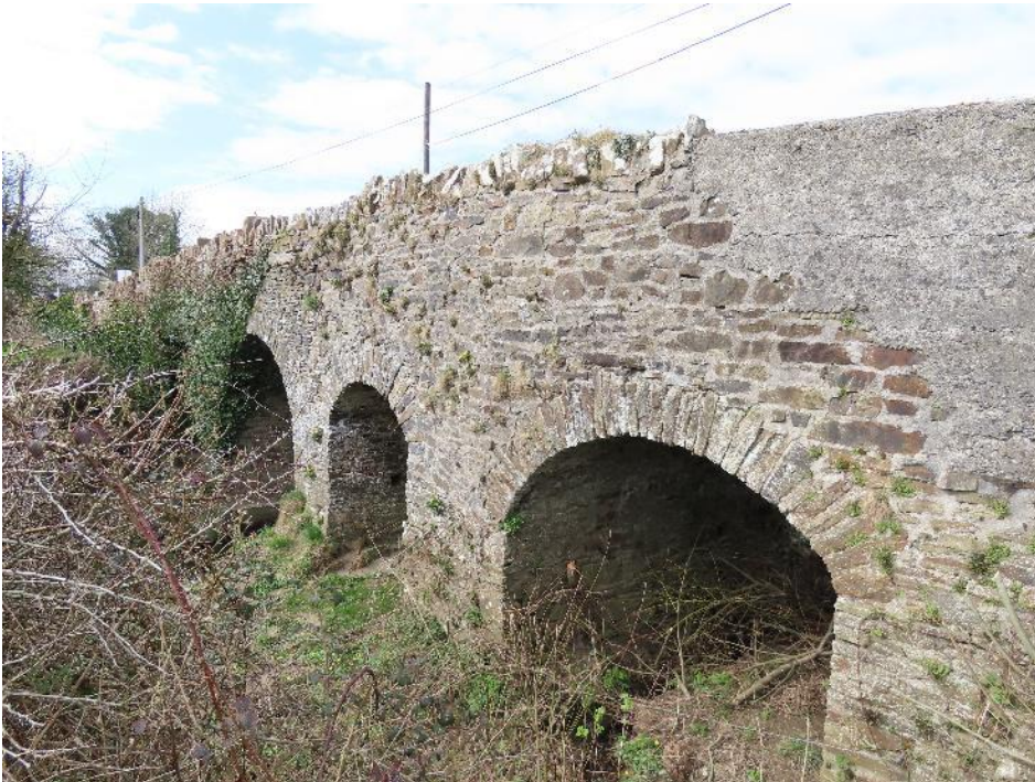
Photo 4 – view across downstream face from eastern side of bridge
