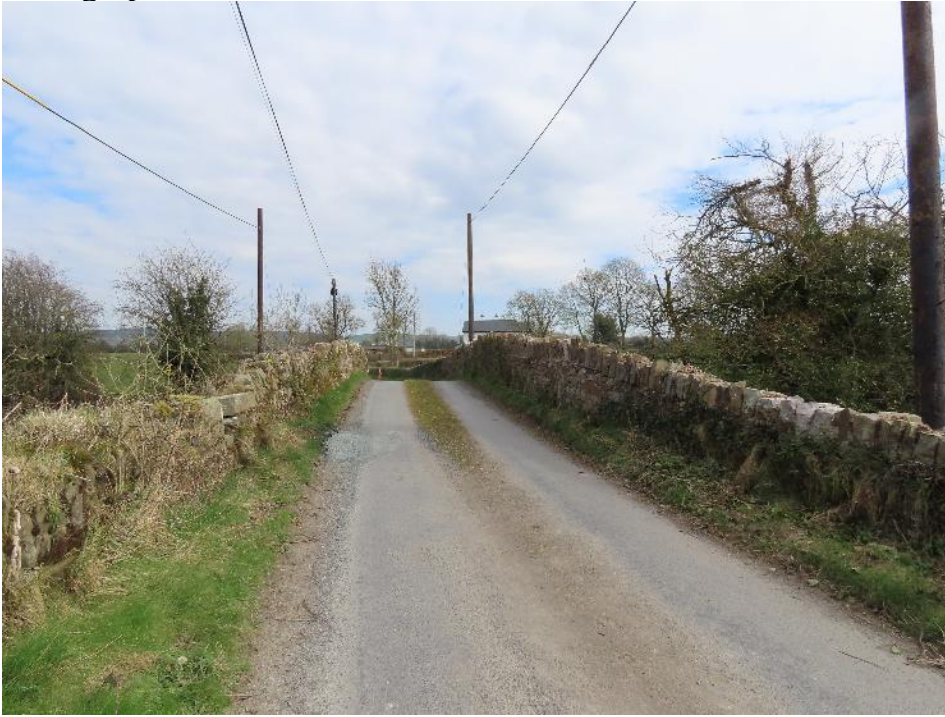
Photo 1 – looking east across Boleybeg Bridge North
