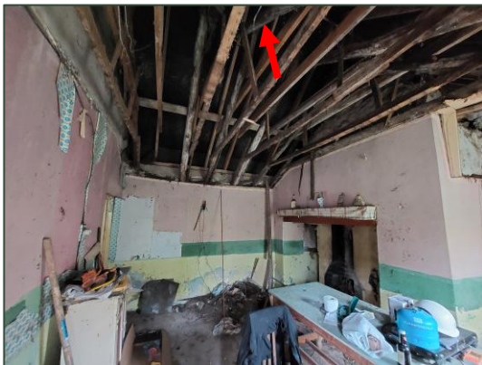
Plate 3.2.6 Interior view of old kitchen, with roosting space on 1 st November 2024 at apex (red arrow). Note the current roof overlaying the previous, older roofing timbers.
