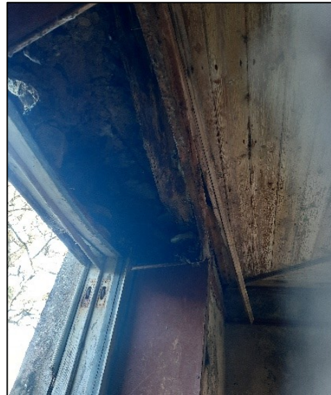
Plate 3-14 Gap between window frame and ceiling.
