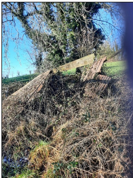
Plate 3-25 Collapsed shed roof with corrugated iron roof and briars covering the structure.
