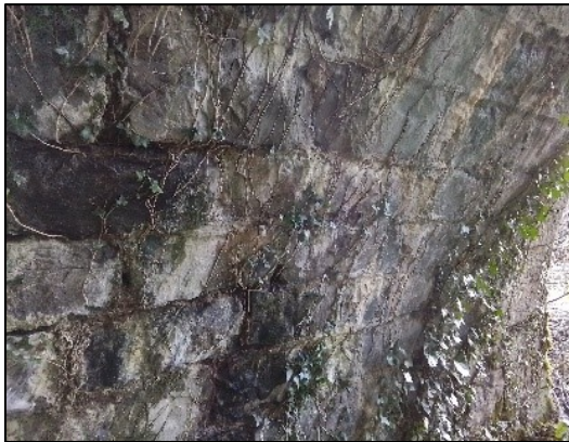
Plate 3-3 Stone blocks are sealed with cement with a small amount of ivy growth, some water leakage through the stonework.
