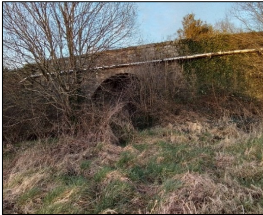
Plate 3-7. Bridge 2 Stone masonry bridge with ivy cover and a pipe along one side.
