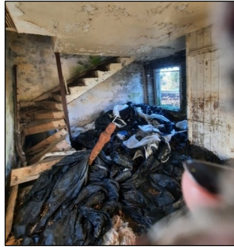
Plate 3-12. Interior view with partially collapsed staircase.
