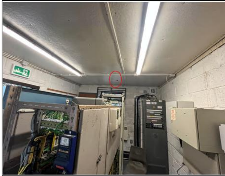
Existing ceiling and gap to be repaired
