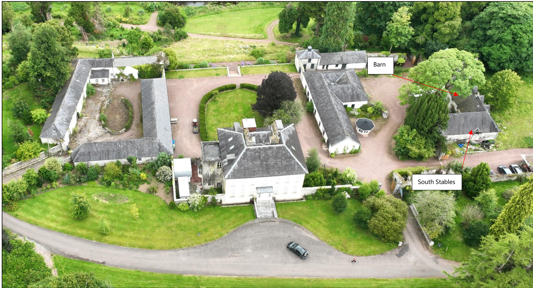
Figure 10: Aerial image indicating location of South Stables and Barn buildings relative to other buildings
