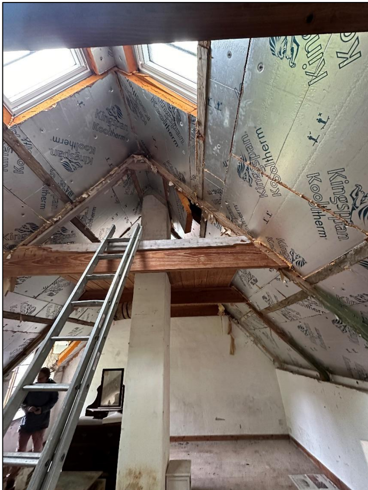
Figure 11: Upstairs room in Barn (which will be retained as is, apart from predator-proofing and segregating space from the lower level of the barn), with colony of bats occurring behind insulation
