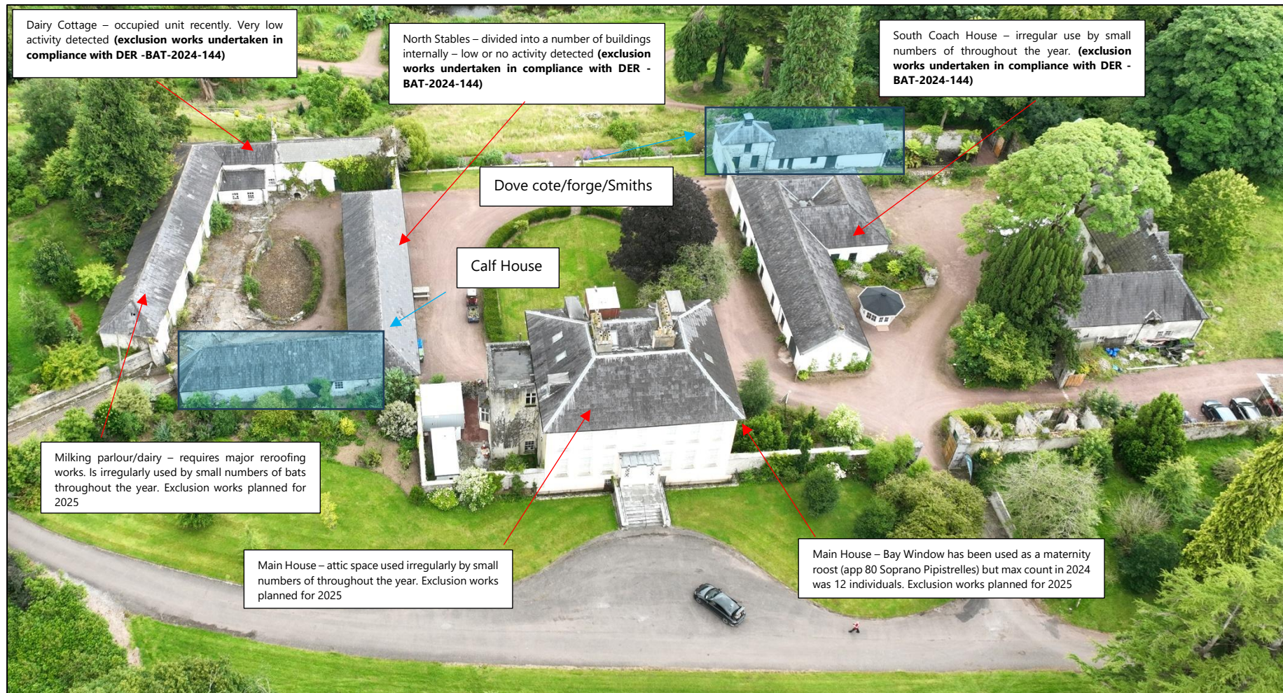
Figure 8: Buildings of limited significance, from which it is proposed to exclude bats (including buildings where exclusion works were undertaken in compliance with DER-BAT-2024-144
