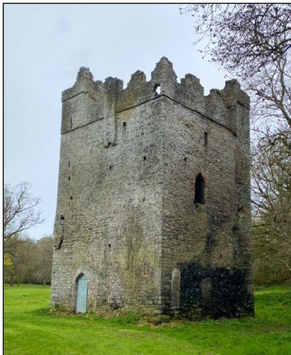
Plate 3: The external northern and western walls of Lanistown Castle
