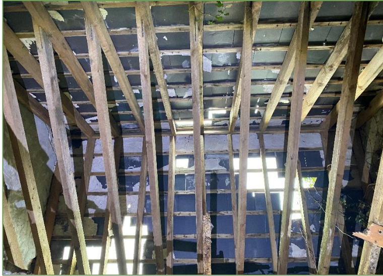
A5. View of the historic roosting location of Lesser Horseshoe Bat within the disused house, showing light and water ingress from missing slates.
