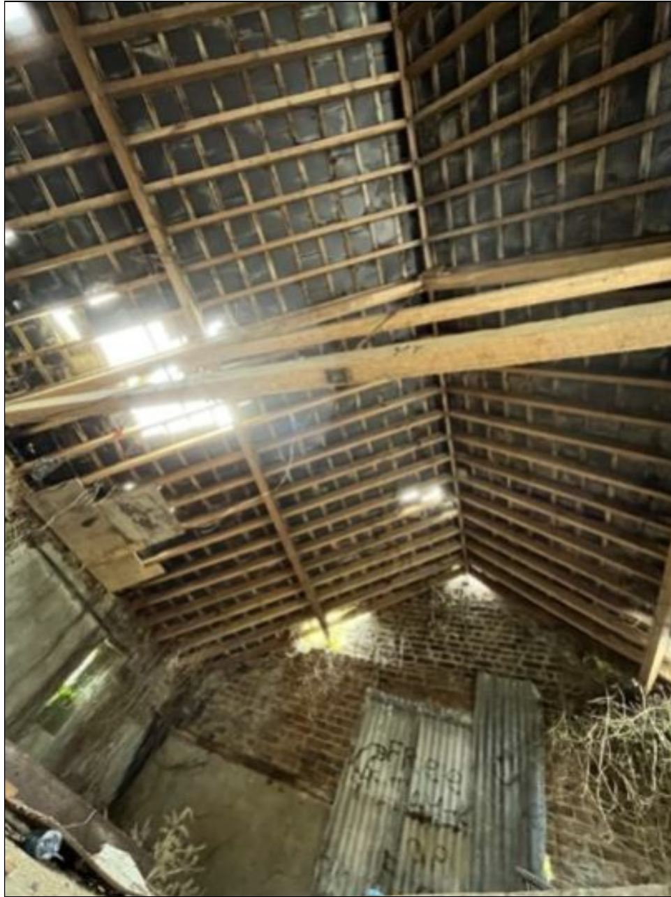
Plate 9. Timber truss of roof.
