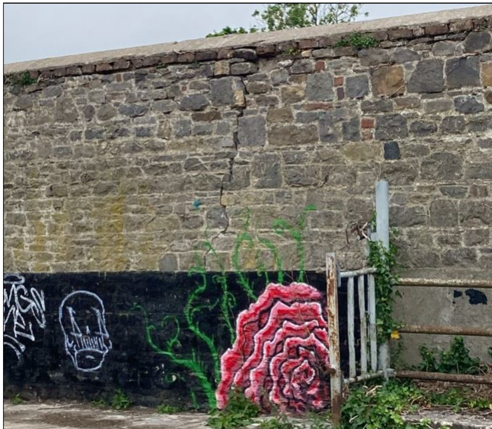
Plate 3. Crack in the NW Wall.
