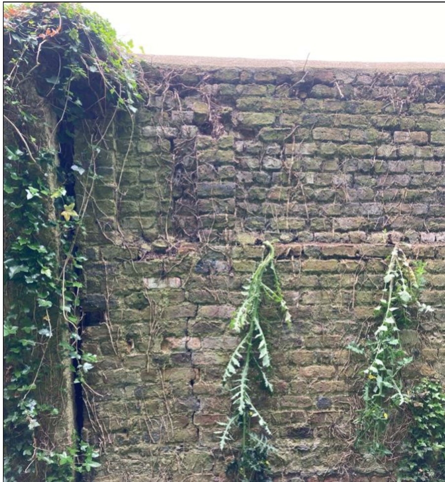
Plate 4. Crack in south-east corner.
