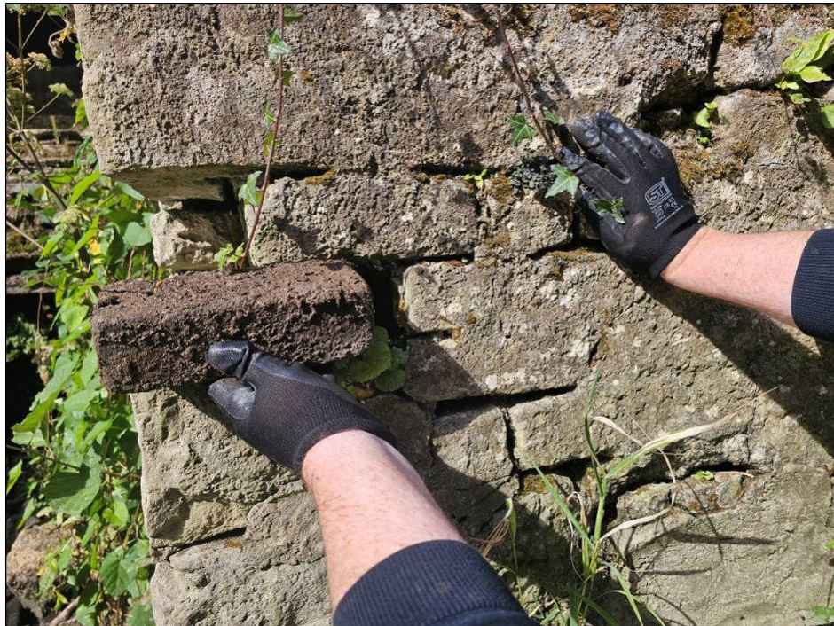
Plate 12. Gaps behind brickwork in the Walled Garden Walls can be created during the stone repairs.
