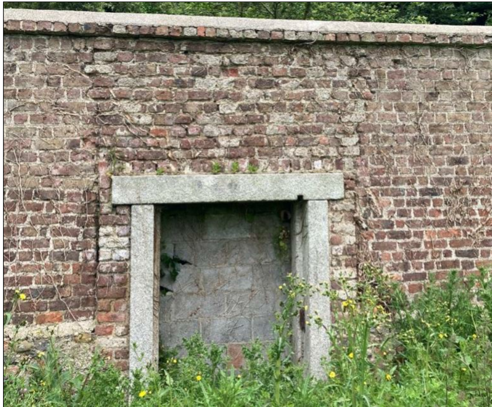
Plate 1. Vertical joint lines at midpoint of Eastern wall.
