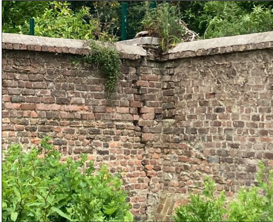
Plate 2. Crack at North-East Corner.
