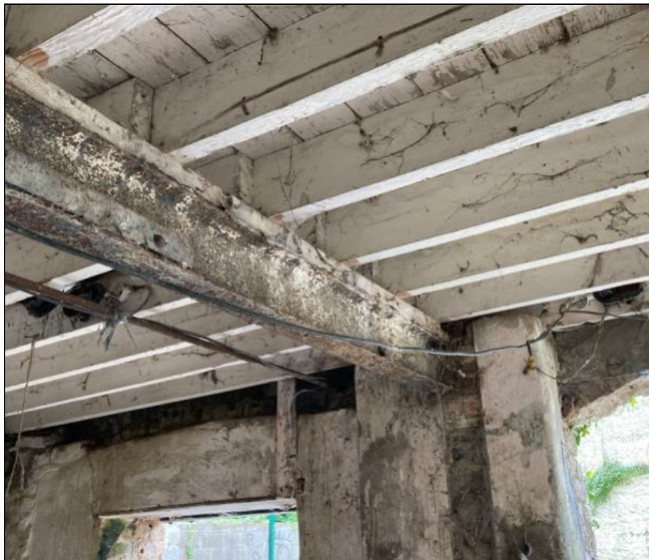
Plate 7. Timber floor joists spliced at steel beam.
