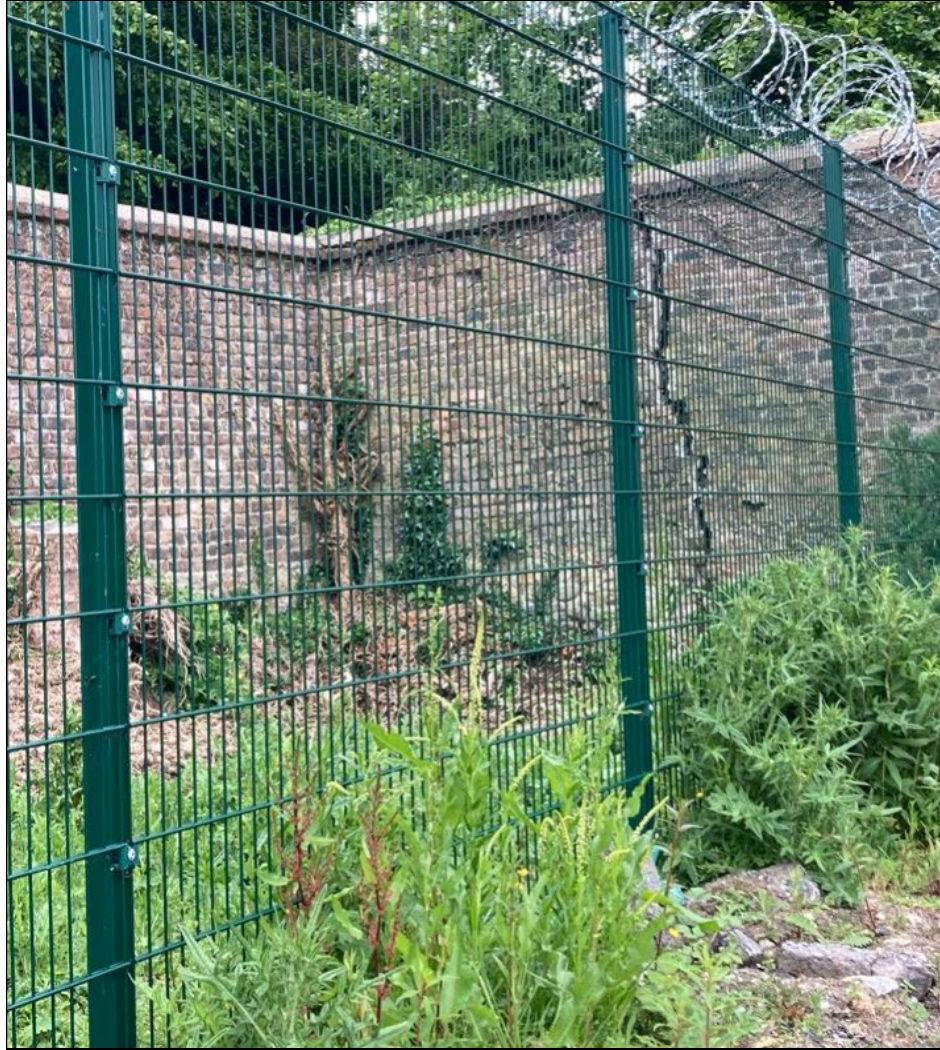
Plate 5. Structural crack in southern wall.
