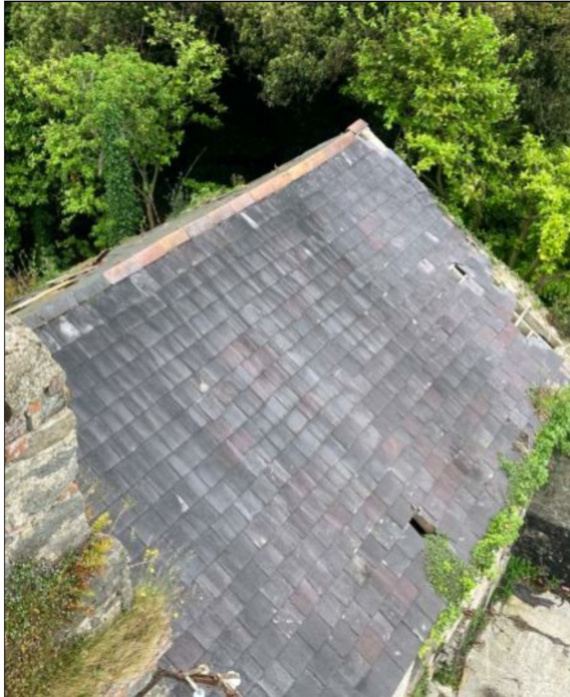
Plate 10. Roof of slate on battens with lime mortar.
