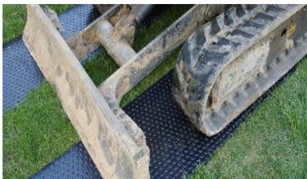
Fig 6 – Ground protection Matting
