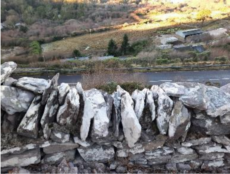
Plate 3. view of upper part of stone wall towards N70
