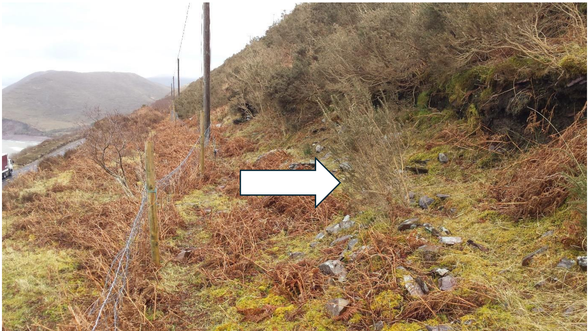
Plate 2: View (i) of loose rock present (Proposed Translocation Site 1).
