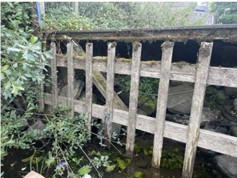
Plate 8: View under jetty in low water level conditions (Source: Traynor Environmental).
