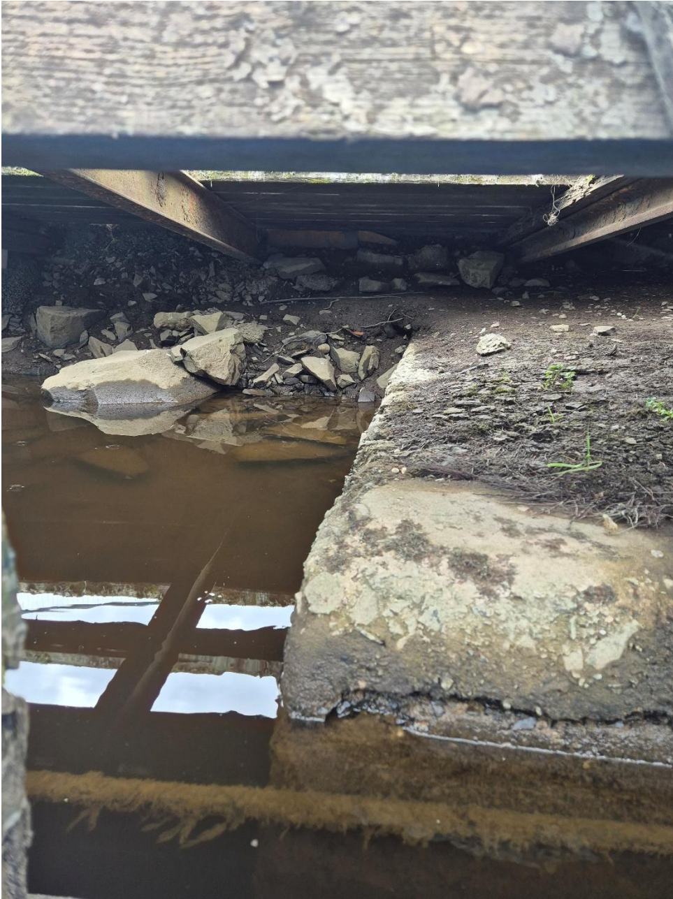
Plate 7: Ducking Stool Jetty, Belturbet, Co. Cavan – view of jetty from river-side during Summer 2026 survey with water levels much lower compared to October 2025 survey.
