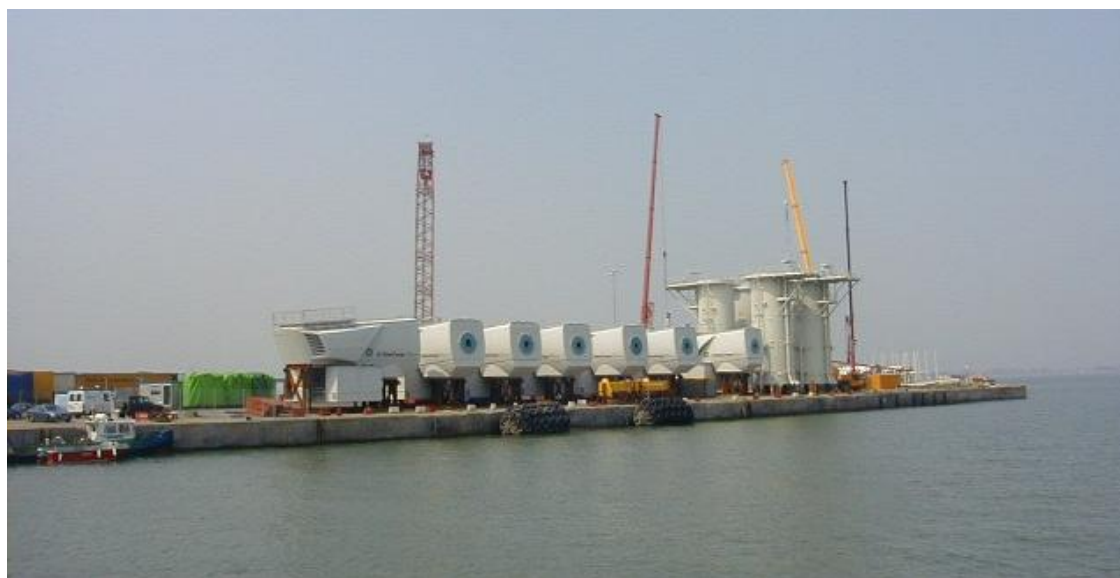
Figure 5-1: Fisherman’s Quay in Rosslare Europort being used for the Arklow Bank Phase 1 project
