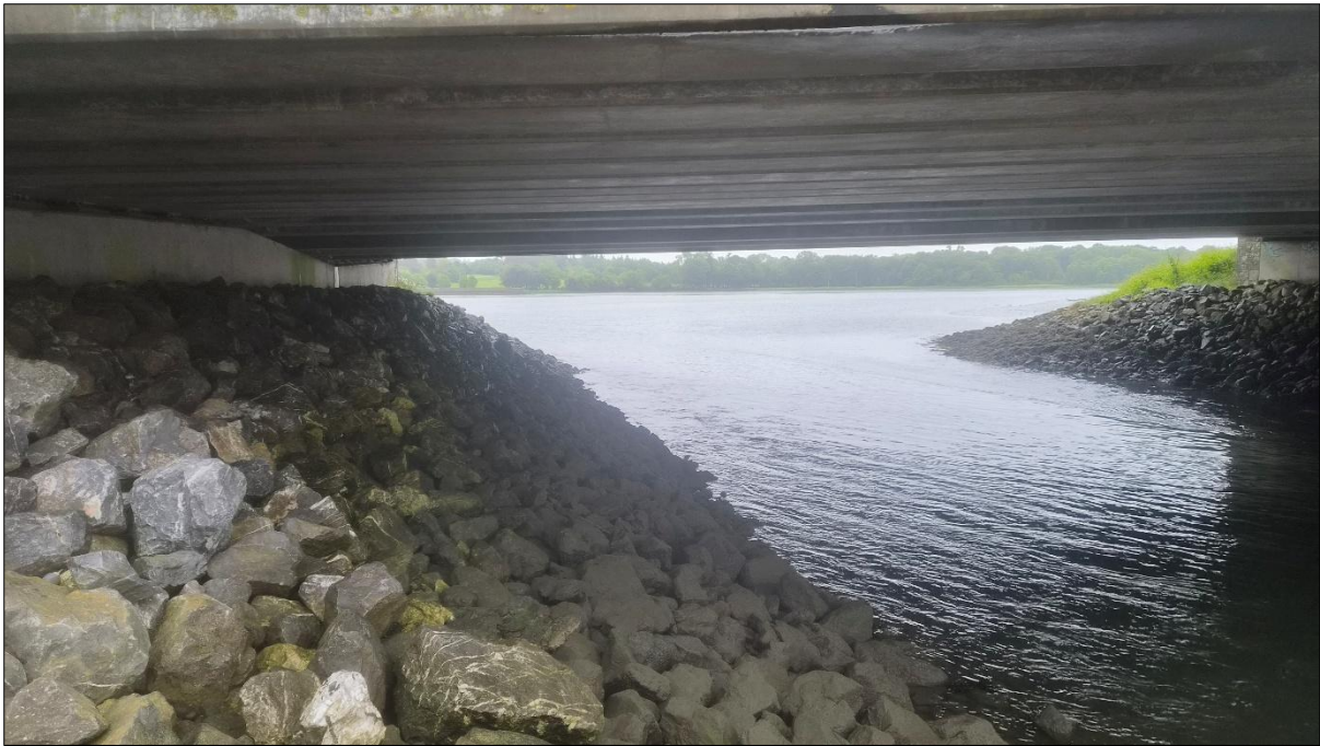
Plate 3.1 N25 Bridge, an area supporting regular otter spraint
