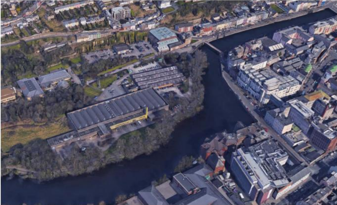
Figure 3.55: Aerial view of North Mall Site
