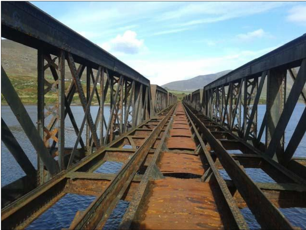
Figure 5. Pre-fabricated steel truss sections will be installed within the existing railway bridge structure
