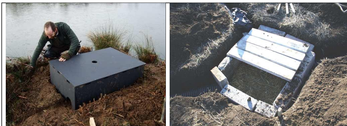
Figure 9. Recycled plastic chamber (L). Constructed chamber with breeze blocks (R). Source: Skinner et al., 2014.
