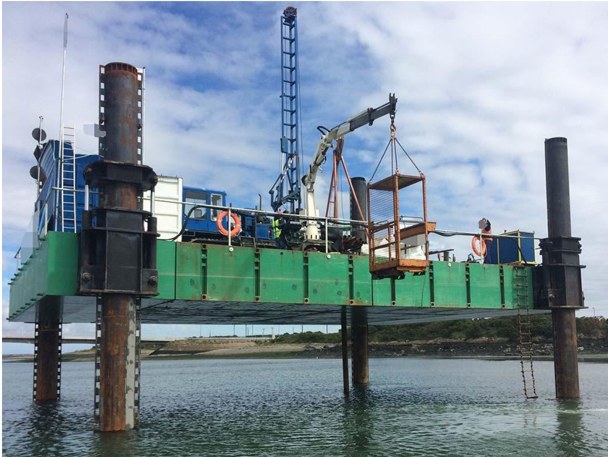
Figure 2-7: Example of a Jack-Up Barge
