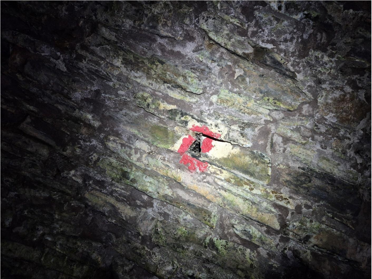
Plate 4-12: Bridge No. 9, Tullyrap, Co. Donegal.
