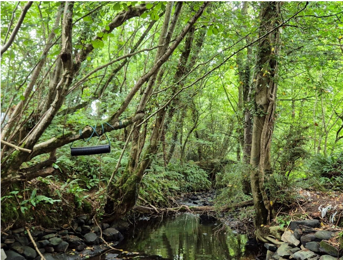
Plate 4-9: Bridge No. 8, Drumbeg, Co. Donegal – vegetation located upstream.
