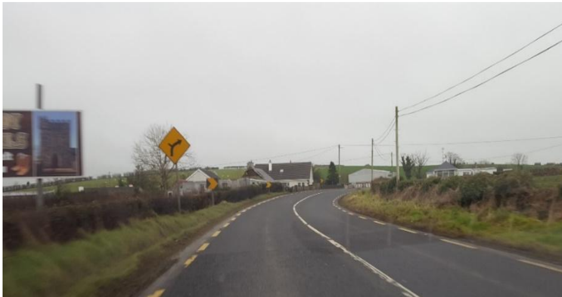
Figure 2.5: N14 Between Manorcunningham and the R236
