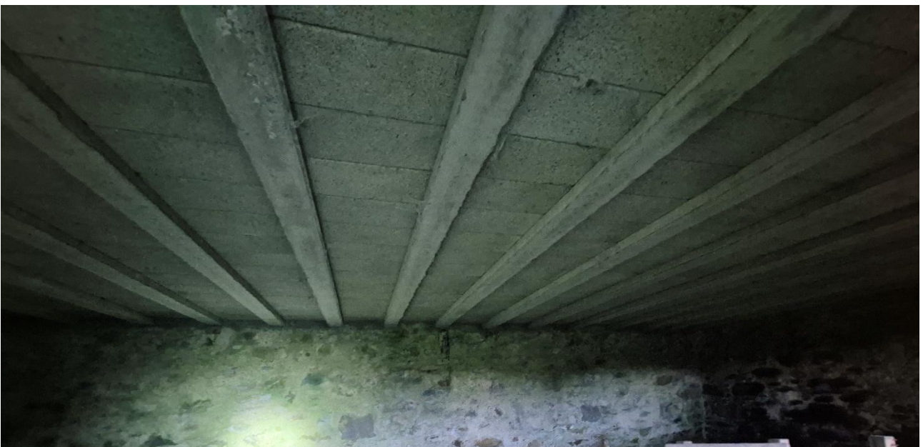
Plate 4-4: Building 1, Pluck, Co. Donegal – internal view, loft floor concrete beams.
