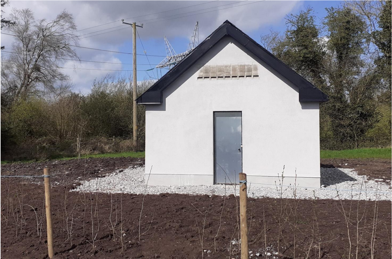
Finished bat house with bat tubes (south facing external wall), Oldstreet Substation Bat House, Co. Galway.
