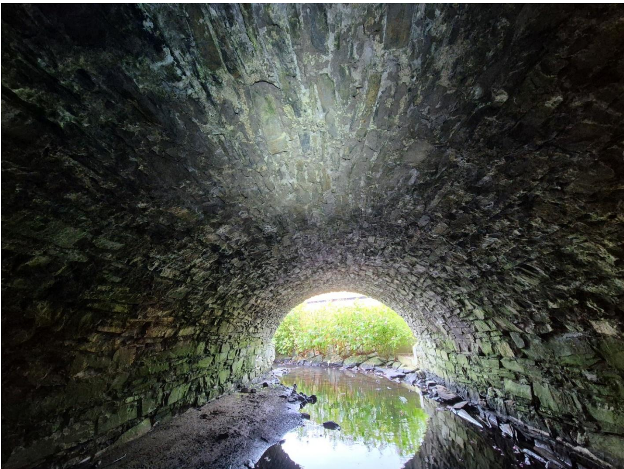
Plate 4-11: Bridge No. 9, Tullyrap, Co. Donegal.
