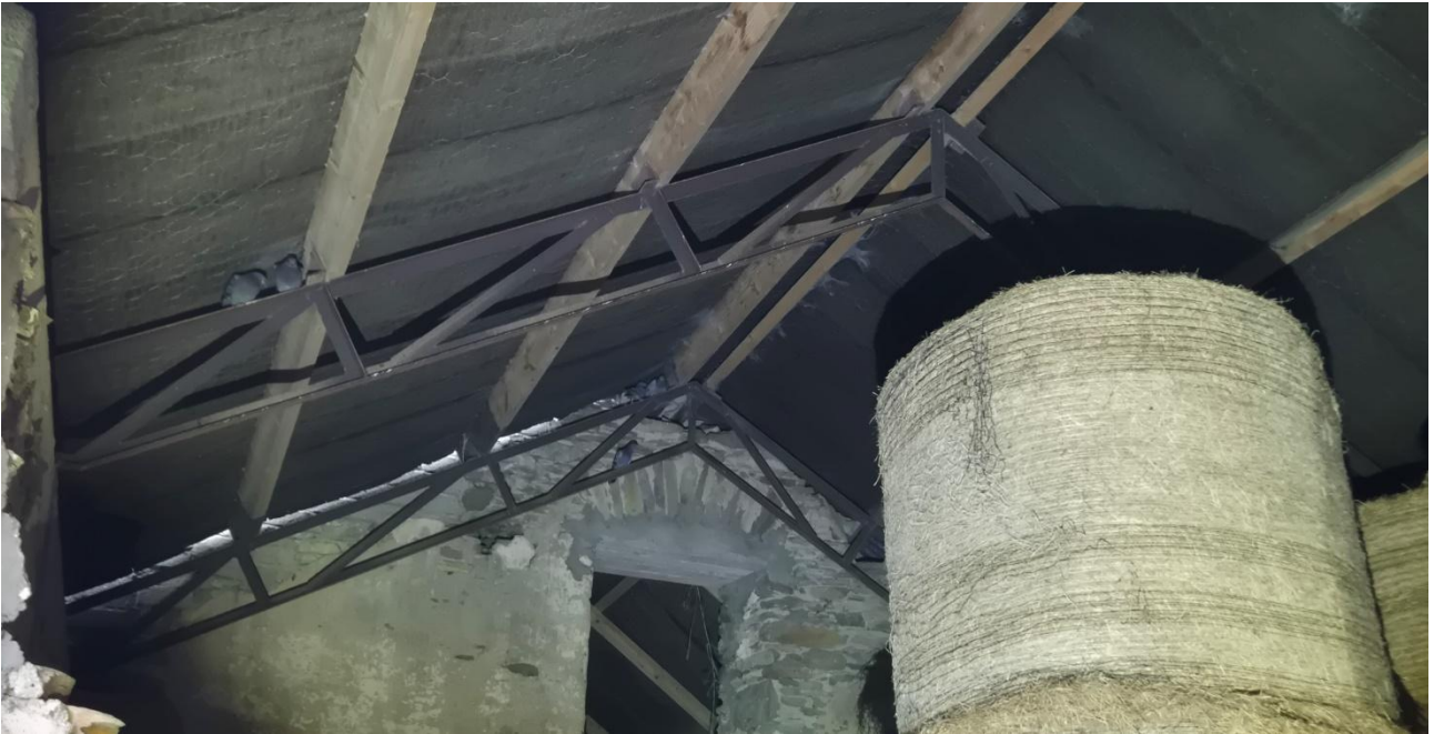
Plate 4-3: Building 1, Pluck, Co. Donegal – internal view.
