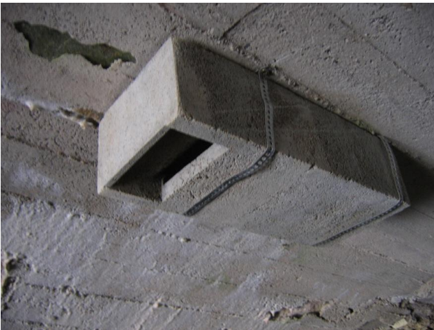
Example of bat tubes fixed to the underside of a culvert and a bat tube built into the external façade of a bridge (Photos: Caroline Shiel and Austin Hopkirk).
