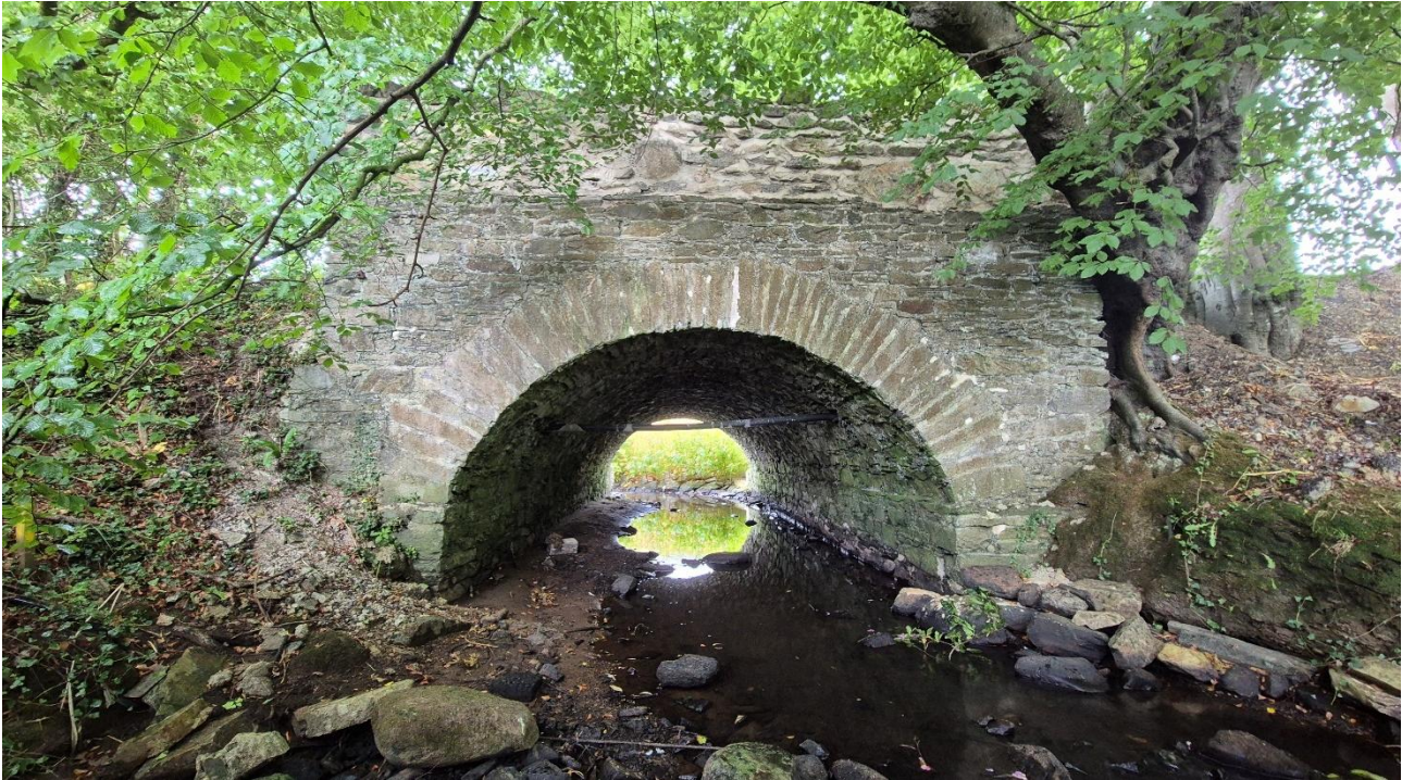
Plate 4-10: Bridge No. 9, Tullyrap, Co. Donegal.
