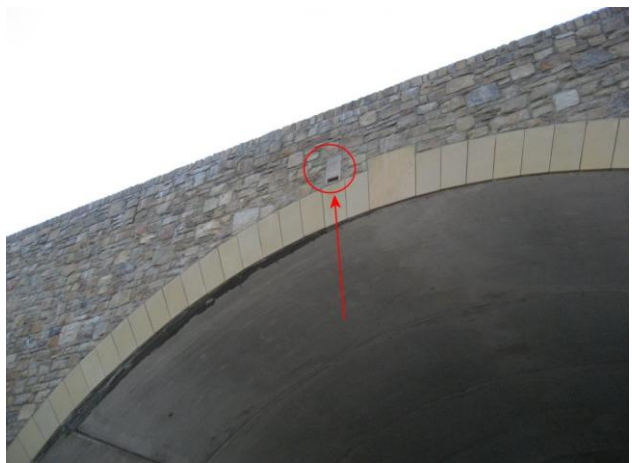
Example of bat tubes fixed to the underside of a culvert and a bat tube built into the external façade of a bridge (Photos: Caroline Shiel and Austin Hopkirk).
