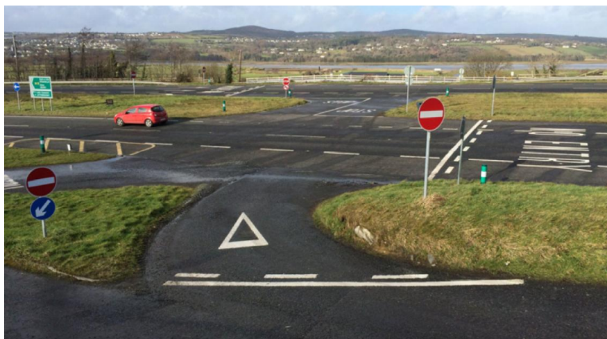
Figure 2.4: Trimragh Junction on the N13 Dual Carriageway
