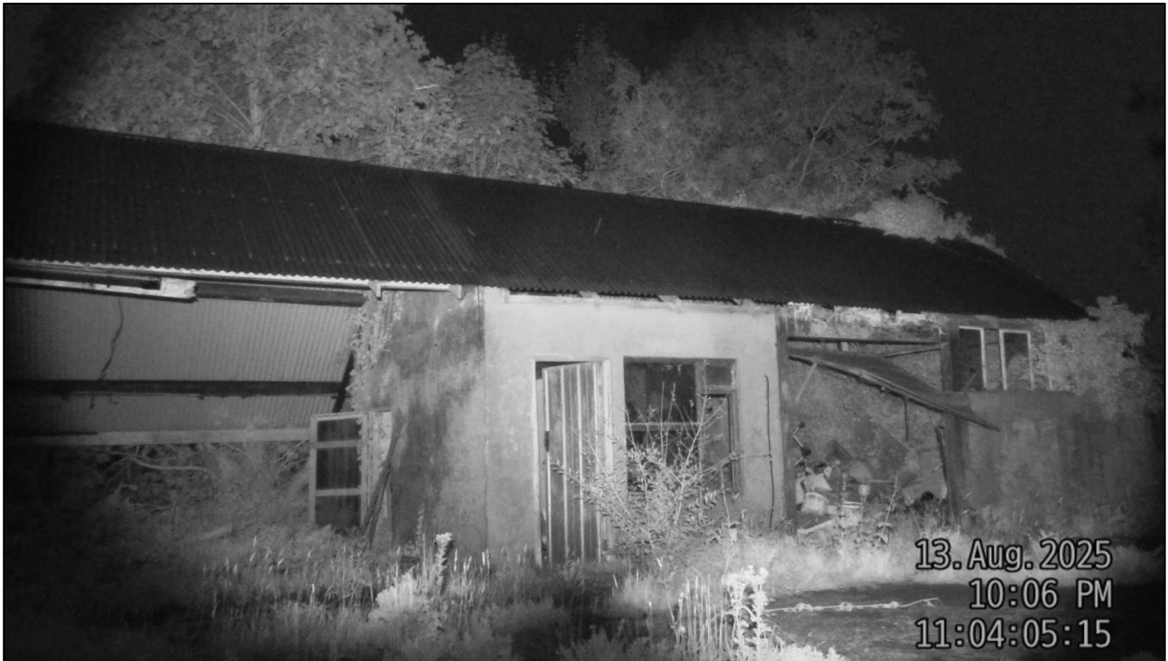
Figure 4-4: Vantage point view of S1 B14b, used on 13 th August and 16 th September
