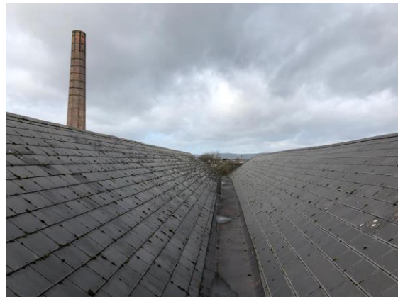
Plate 2 Central roof valley, intact slate work.
