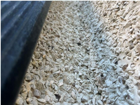
Plate 5 Bat droppings on spiderweb beneath west apse soffit north elevation
