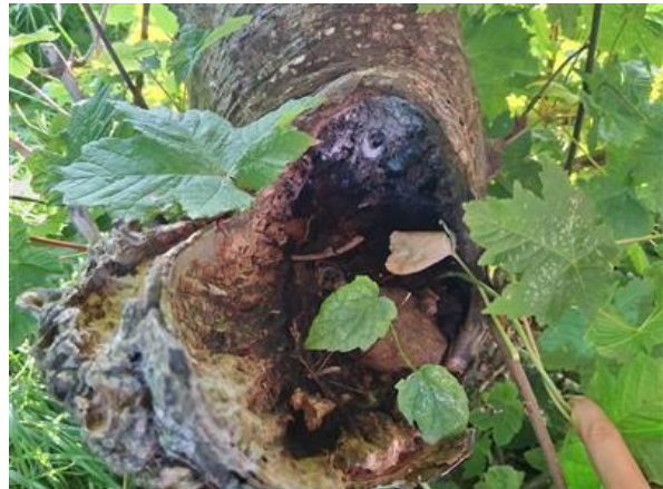
Plate 18 Tear out within sycamore tree on NE boundary
