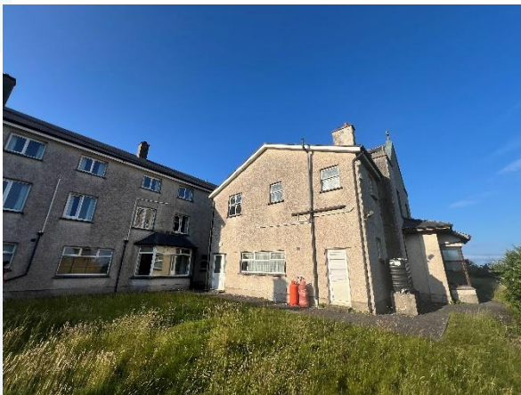
Plate 3 Southwest elevation of convent
