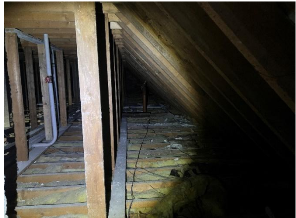
Plate 12 1923 convent attic showing no evidence of bats.
