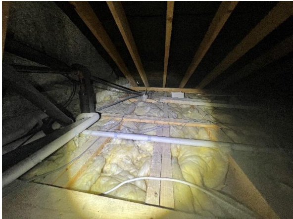
Plate 13 1923 convent attic showing no evidence of bats.
