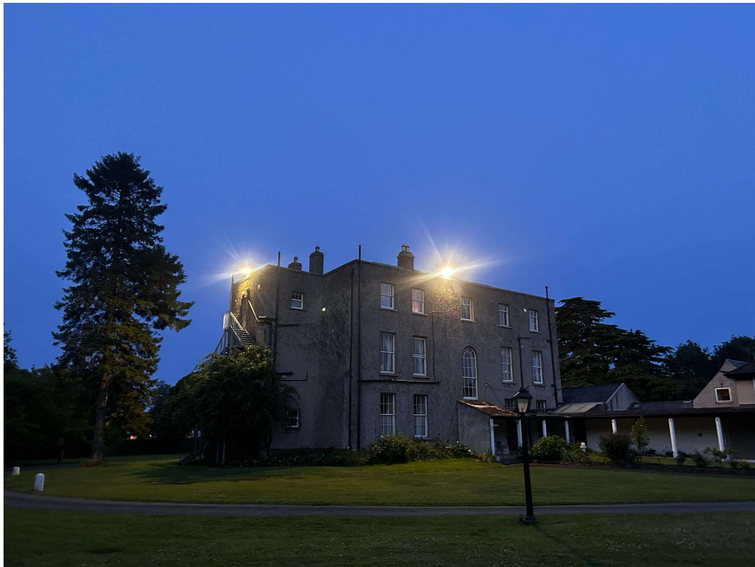
Plate 1. Main building on site proposed for retention and refurbishment (courtyard buildings to the rear to be demolished)
