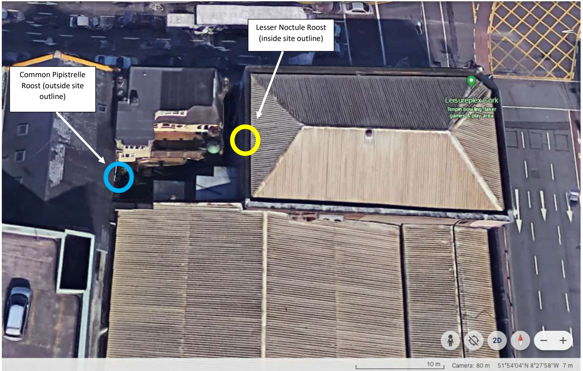
Figure 13. Location of bat roosts onsite (Lesser Noctule roost = yellow circle) (Common Pipistrelle roost = blue circle) (Source: Google Earth 3D)
