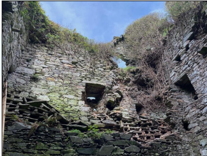
Plate 3 Internal western wall of the castle where works are proposed
