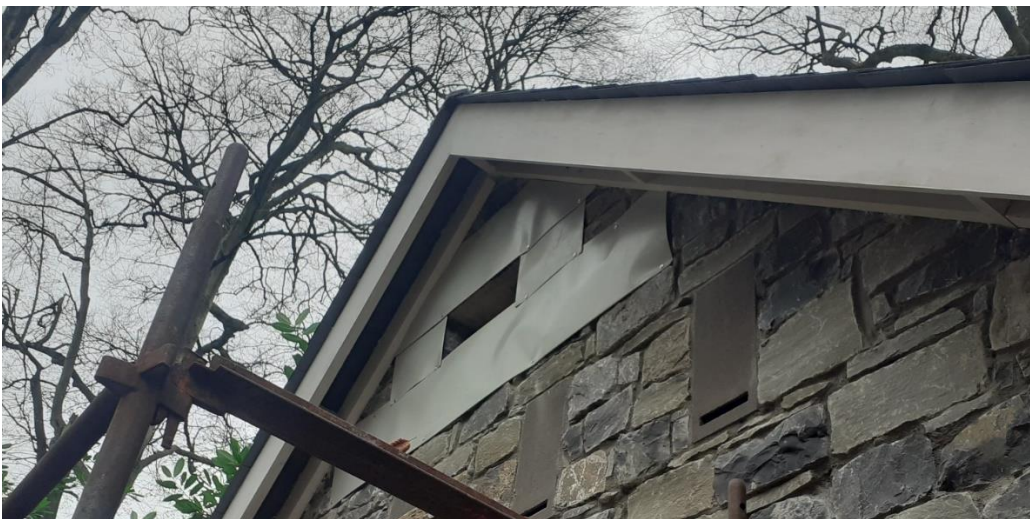
Plate 6: Example of predator proofing on external wall around entrance point of bat house.
