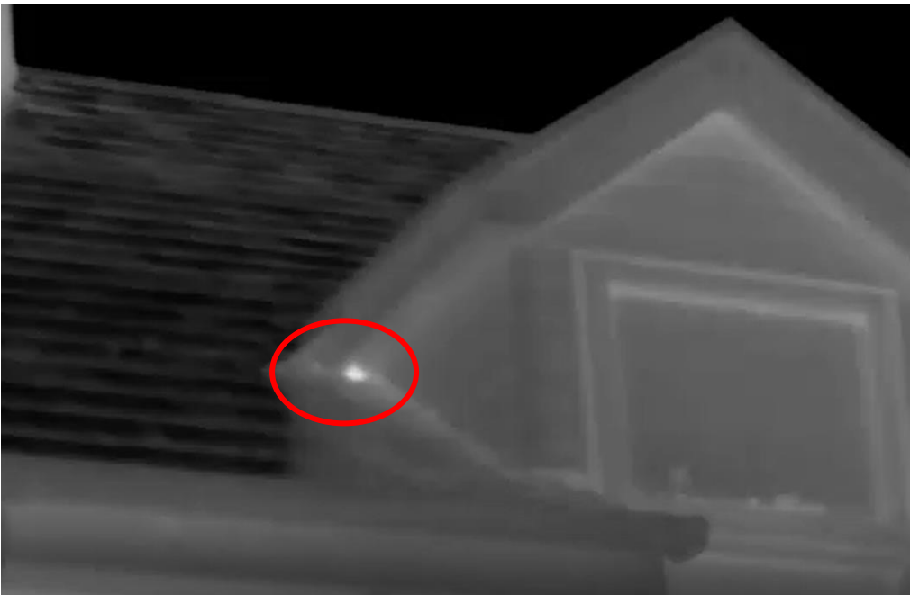
Plate 5: Screenshot of thermal imagery filming of common pipistrelle roost exit point of the front dormer window of Building 2 (bright section – emerging bat).
