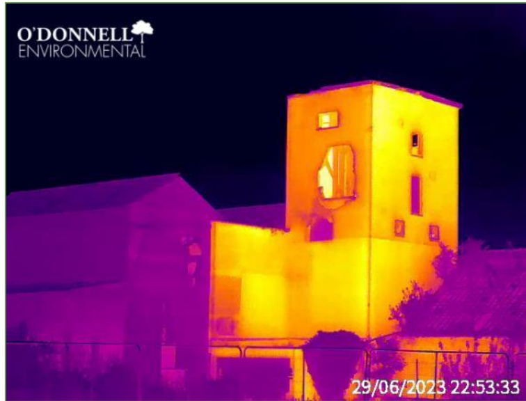
Plate 2.6 Example image from thermal camera covering the eastern aspect of the former mill buildings complex.
