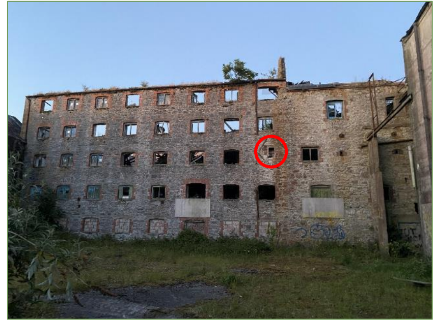
A12. View of the western aspect of the mills building complex, with location of Kestrel nesting site within old fireplace (red circle).
