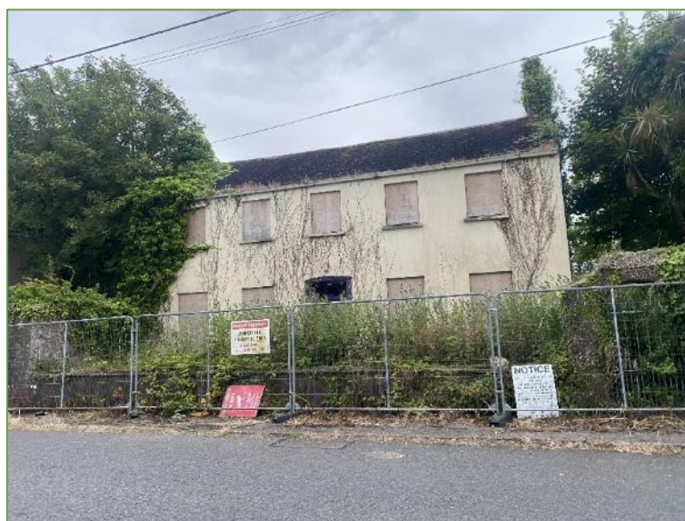
Plate 3.2.2 View overlooking the northern/front aspect of Eastville House from the adjacent roadway (L3625).
