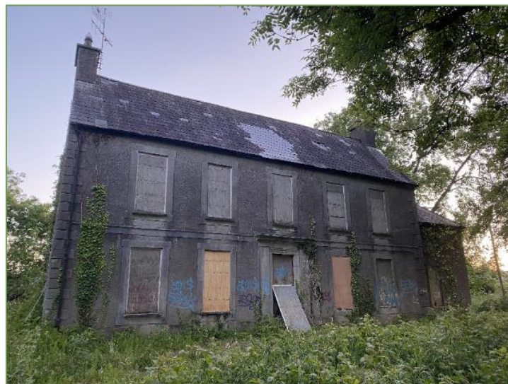
Plate 3.2.1 View overlooking the eastern/front aspect of Roseville House.
