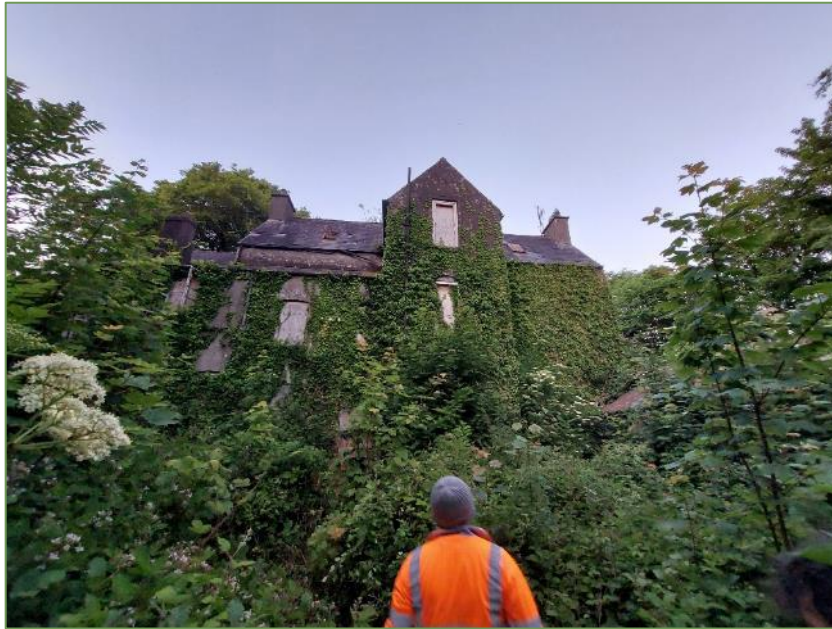
A5. View of the western aspect of Rosehill House.
