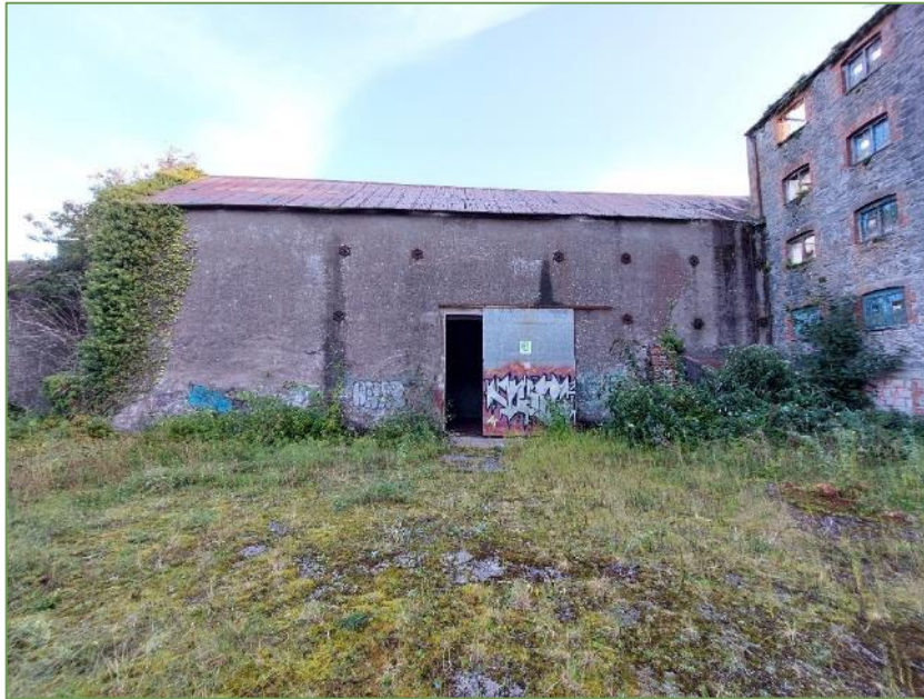
A3. View of the stonework grain store within the mills complex.
