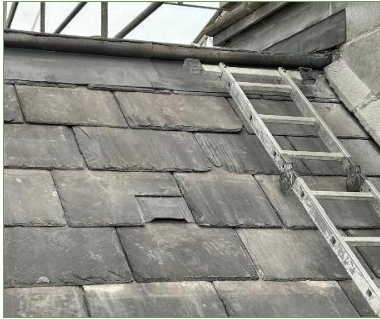
Plate 5.2 - Example of a lead bat access tile (Photo: Tom O'Donnell).
