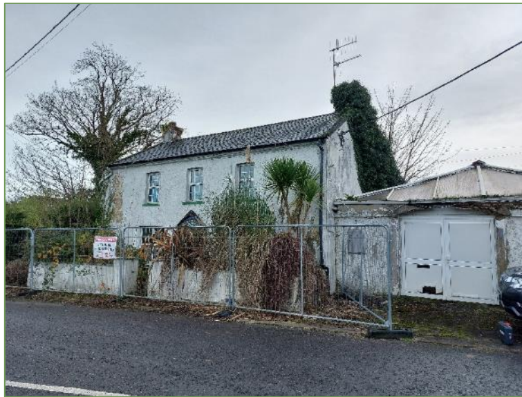
Plate 3.2.5 View overlooking the northern aspect of the former residence.
