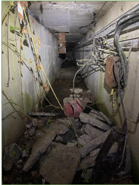
A13. View of the underground tunnel network within the development site.
