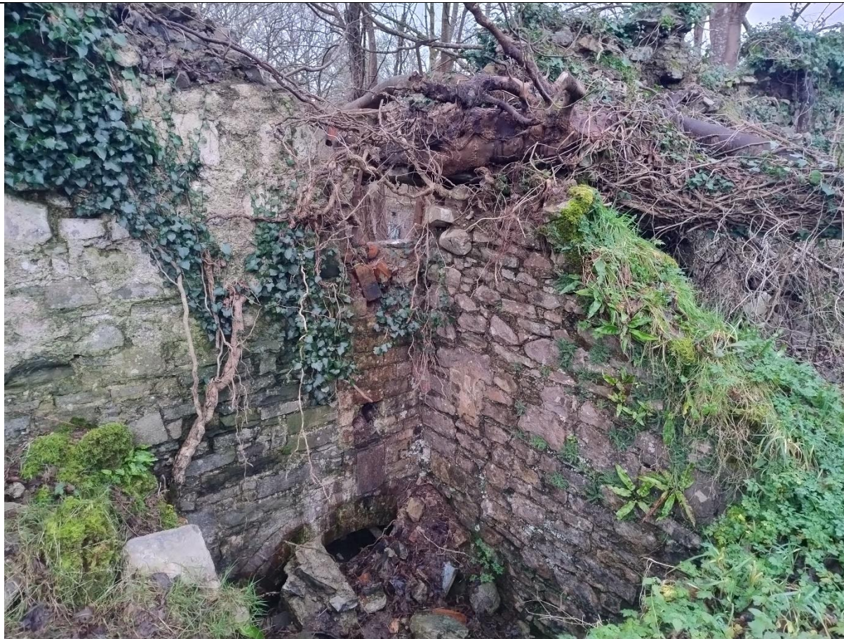
Figure 4: Brick store. Pipistrelle recorded in crevice. Hibernacula damaged by falling tree during storm Eowyn.
