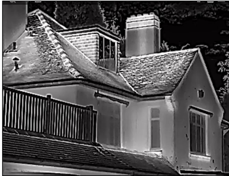
FIGURE 3. EXAMPLE OF THERMAL IMAGAGING CAMERA FOOTAGE CAPTURED DURING EMERGENCY SURVEYS.
