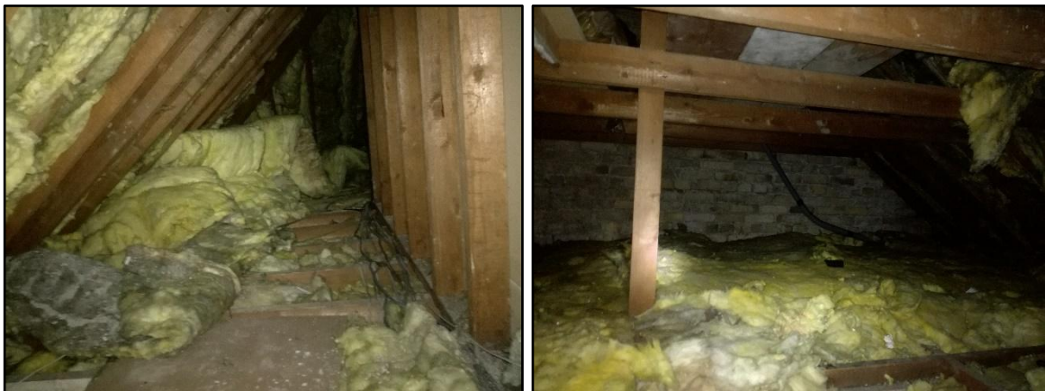
FIGURE 7. ATTIC SPACE OF EXISTING BUILDING.
