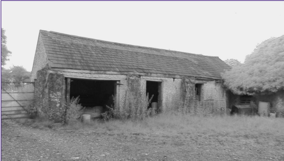
Plate 1: (2023) looking North at Structure (S1) at beginning of survey.
