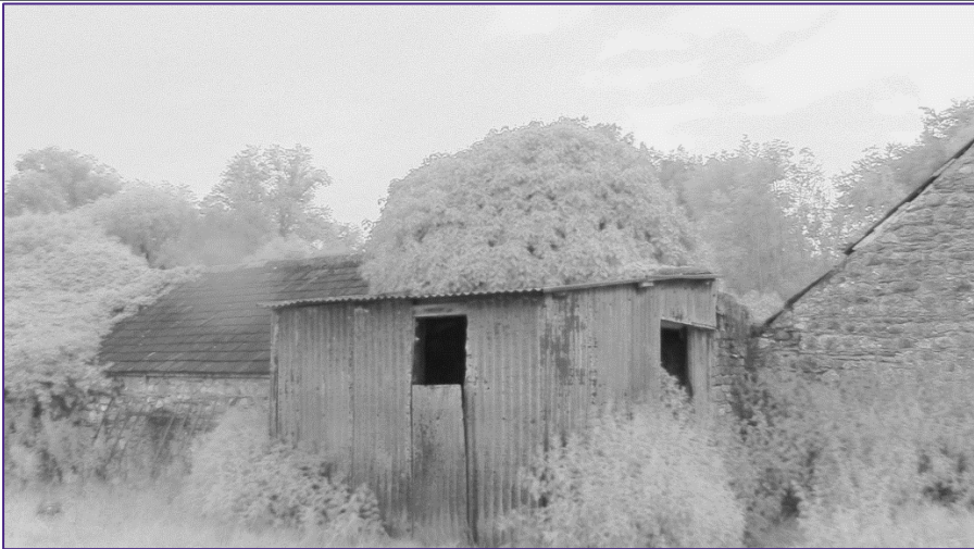
Plate 9: (2023) Looking West at Structure 2 (S2).
