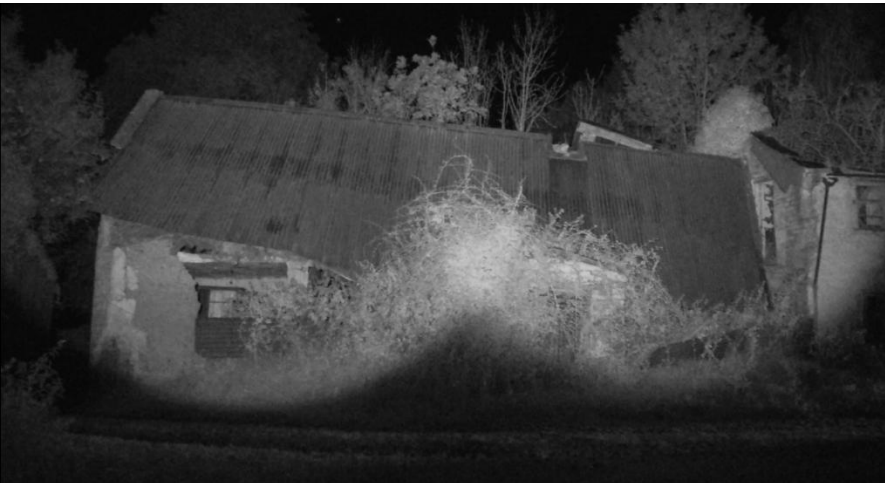
Plate 23: (2025) Looking West towards Structure 4 (S4) during the darkest part of the survey
