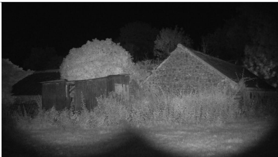
Plate 13: (2023) Looking West at Structure 2 (S2) and Structure 1 (S1)
