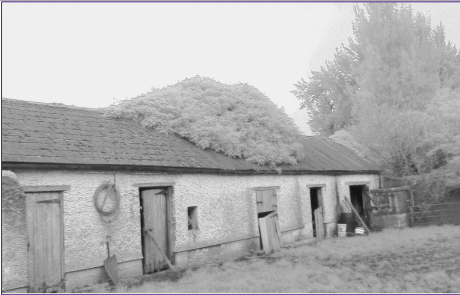
Plate 7: (2023) Looking Southwest at Structure 2 (S2) at beginning of survey.
