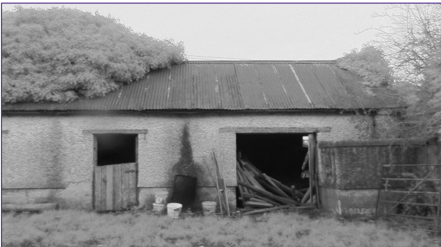
Plate 10: (2023) Looking East at Structure 2 (S2) at beginning of survey.
