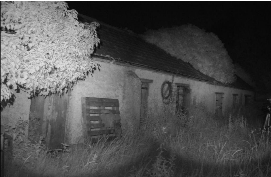
Plate 12: (2025) Looking east at Structure (S2) during darkest part of the survey.
