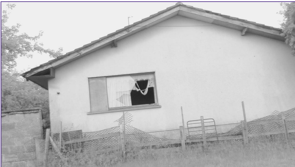
Plate 29: (2023) Looking West at Structure 6 (S6) at the beginning of the survey.
