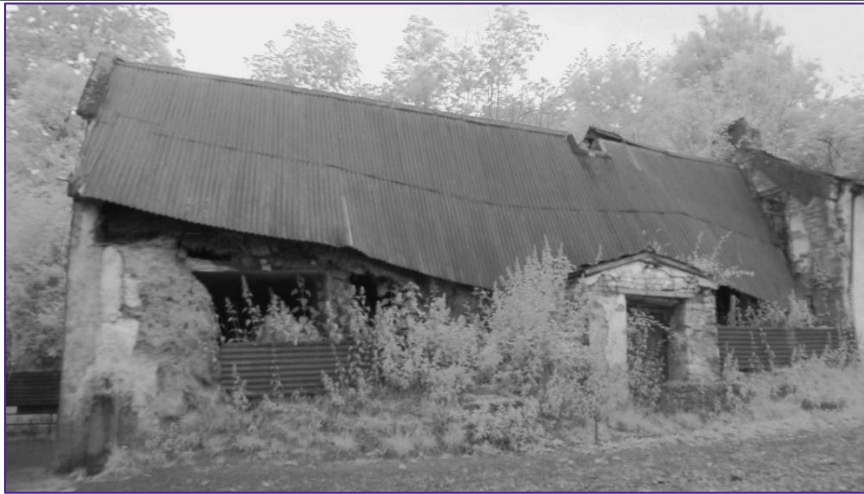
Plate 20: (2023) Looking West towards Structure 4 (S4) at the beginning of the survey.
