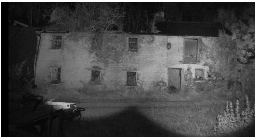
Plate 19: (2025) Looking West towards Structure 3 (S3) during darkest part of survey
