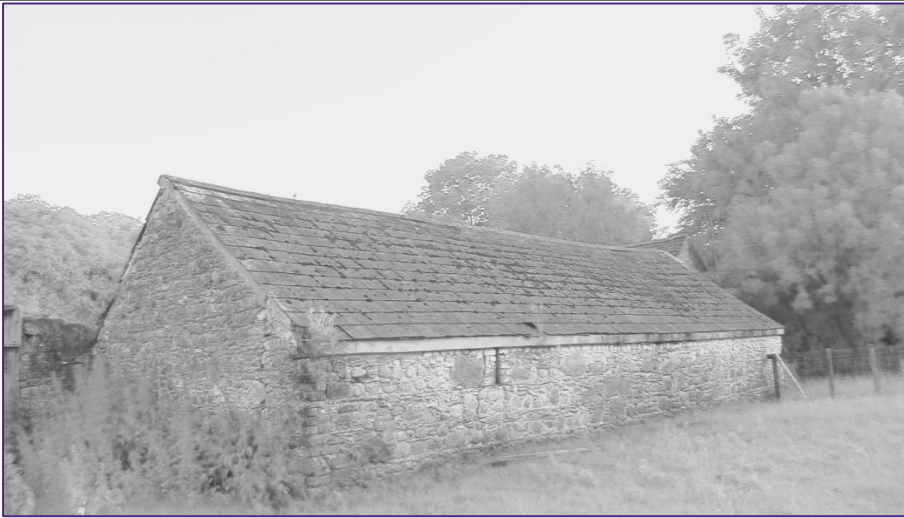
Plate 3: (2023) Looking Southwest at Structure 1 (S1) at beginning of survey.
