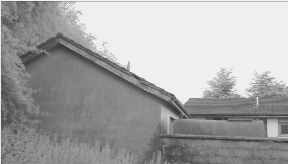
Plate 26: (2023) Looking North at Structure 5 (S5) at beginning of survey.
