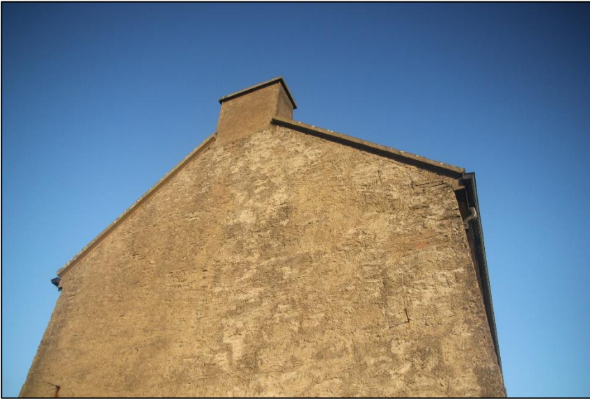
Plate 4 Other side façade also well sealed.
