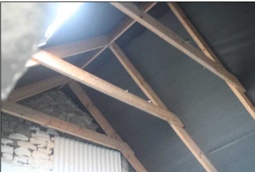
Plate 15 First barn with numerous barn swallow nests and fledging's. Also contained bat droppings on walls.
