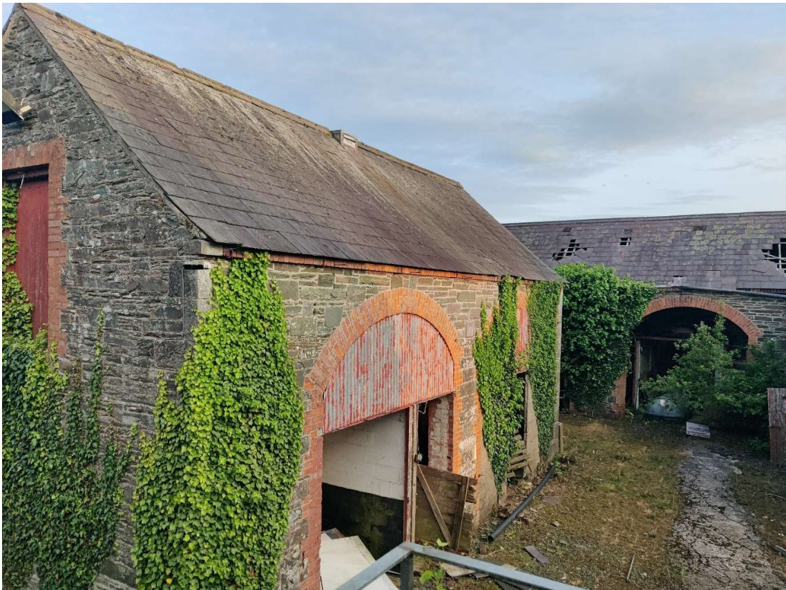
Plate 6. Courtyard stable structure
