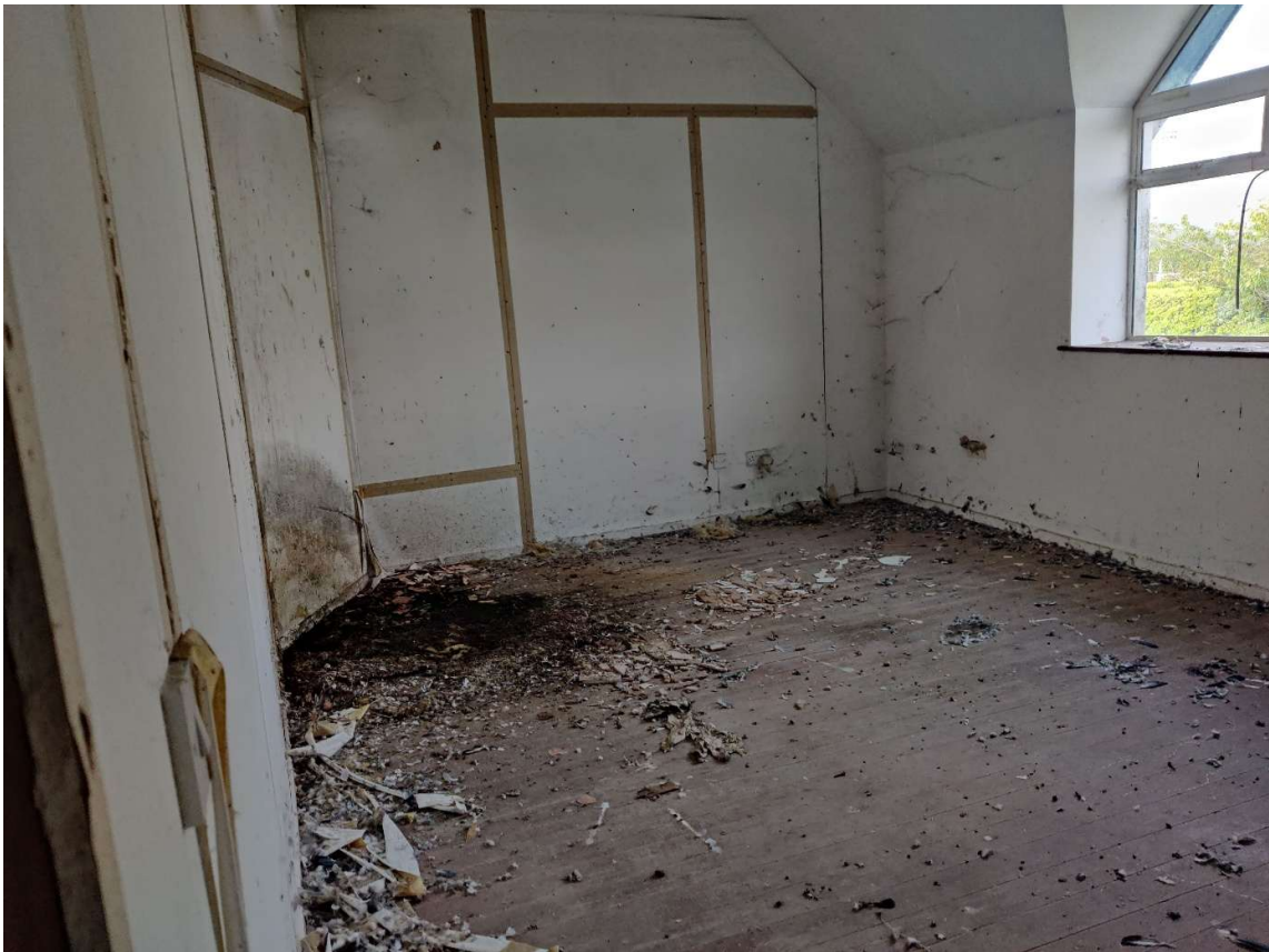
Plate 3. 2 nd Storey of RIC Stable building
