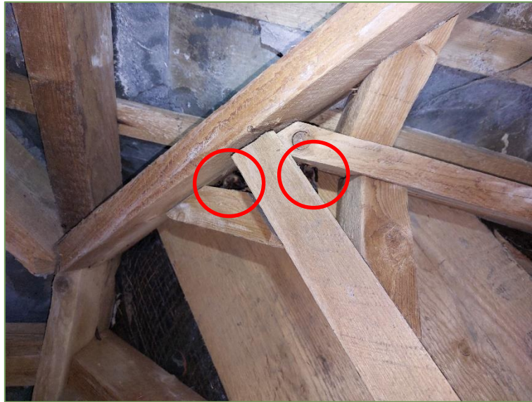
Plate 3.2.7 Two Brown Long-eared Bats (red circles) located within the joinery apex of the western attic section of the former Garda Station
