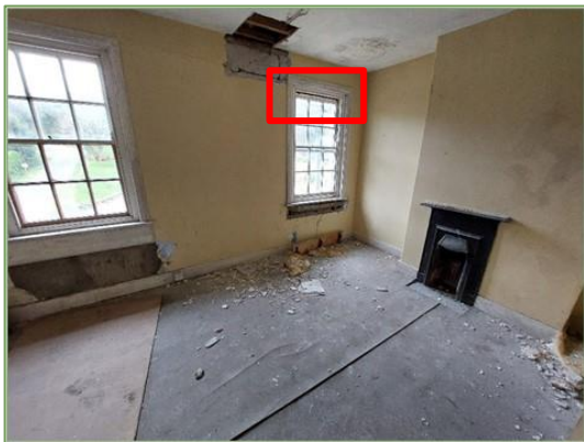
Plate 3.2.3 View of the upper floor room with open sash window (red box).
