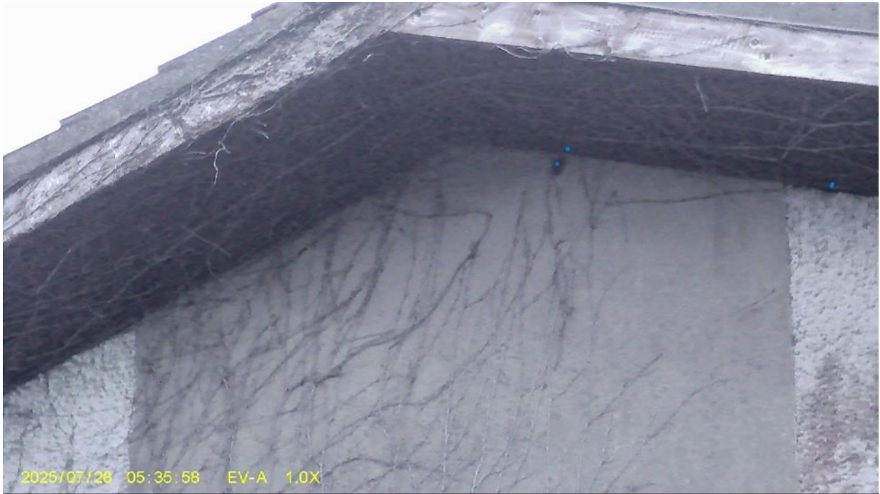
Plate 5. Soffit gap to be retained during supervised replacement works.
