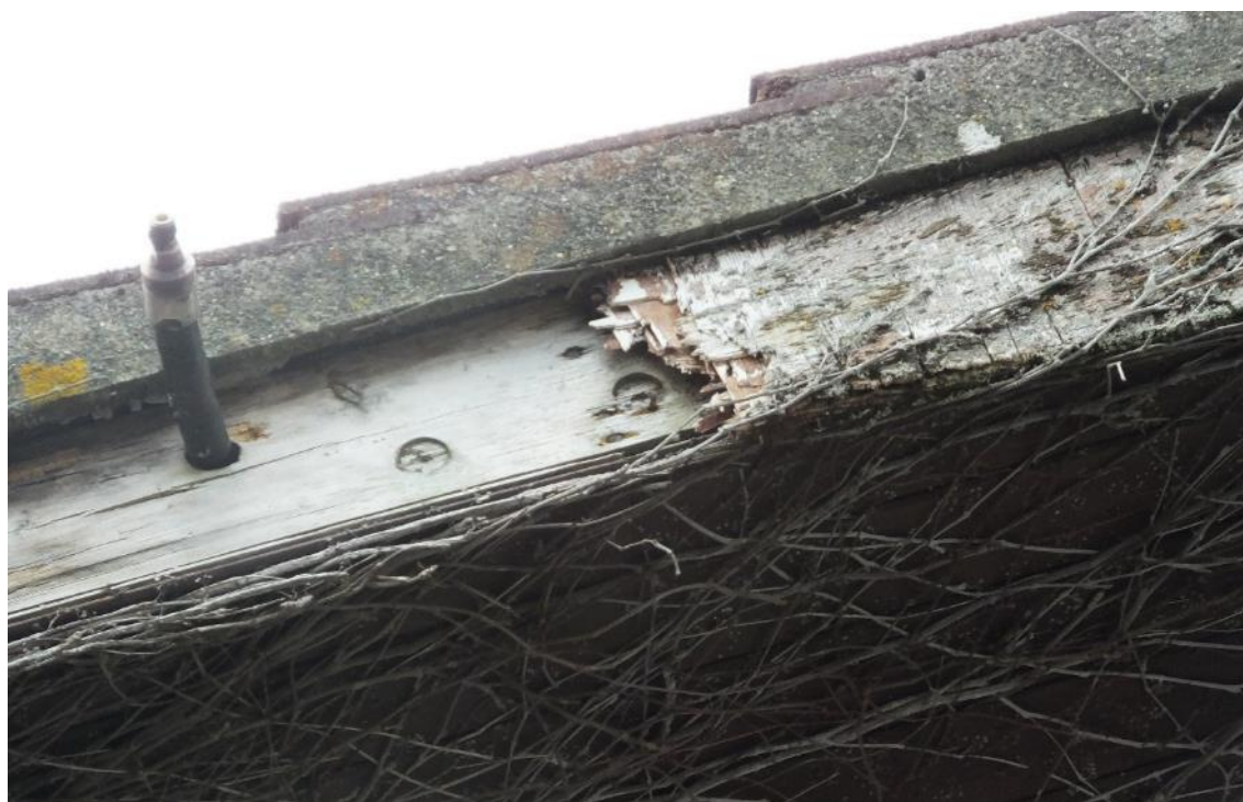
Plate 15: South facing fascia is weather worn and has potential to host bats
