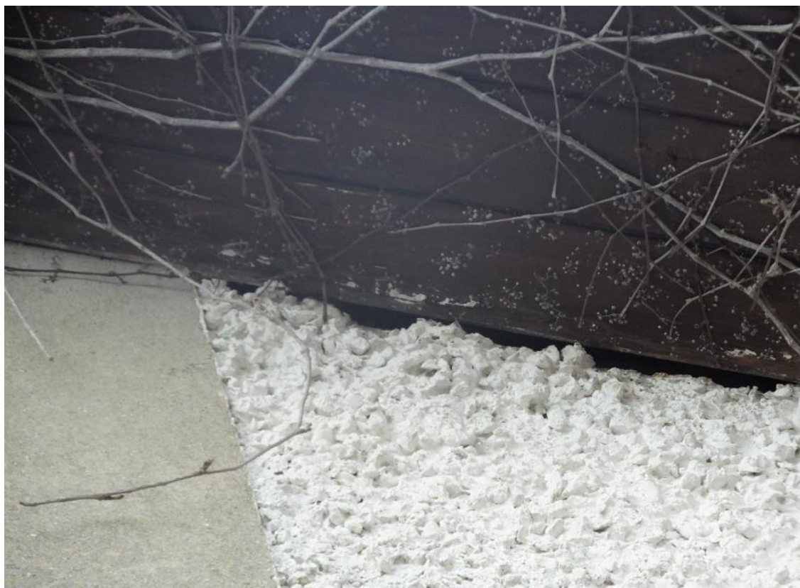
Plate 14: Some gaps in the eaves appear large enough for bats to enter at south end (1)
