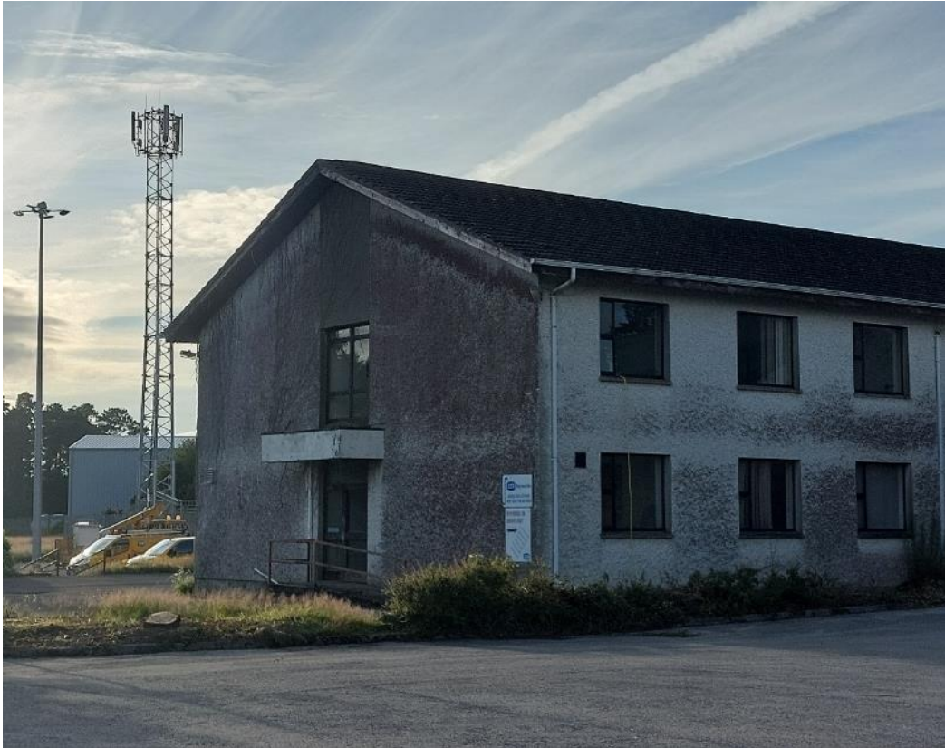
Plate 8: South end of main building (1)
