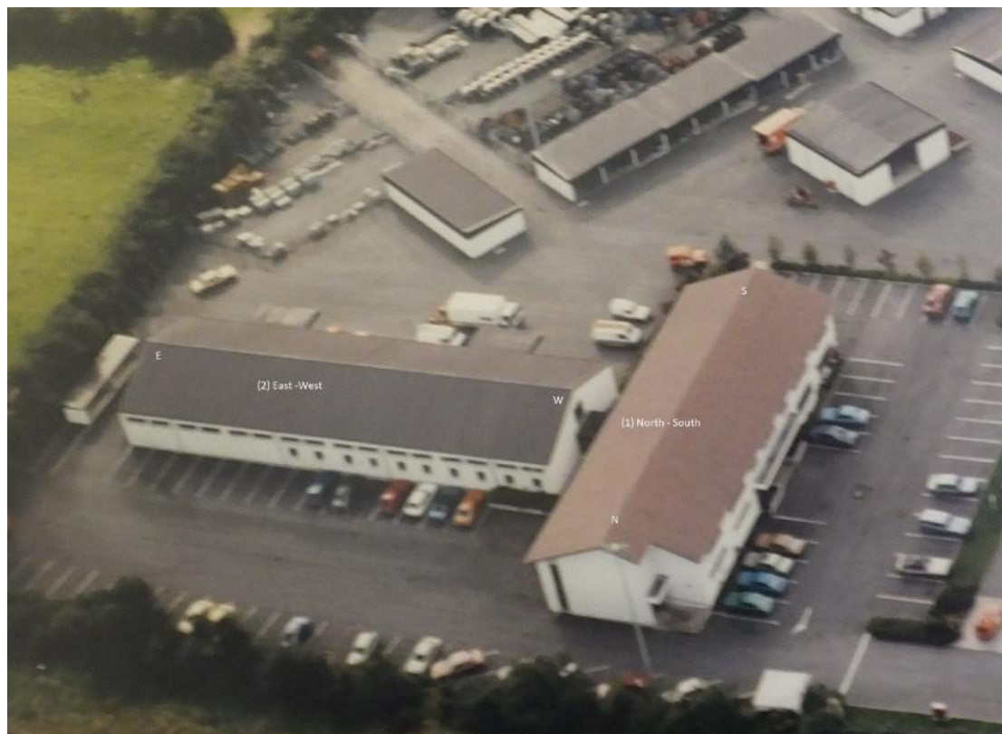
Plate 1: Aerial view of T-shaped office building (1), North – South and (2) West – East
