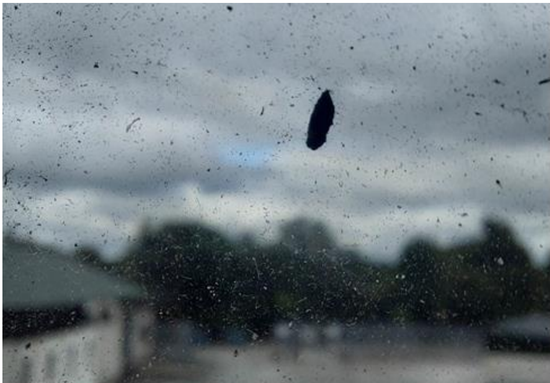
Plate 13: Bat dropping on outside of windowpane at the south end of building (1)
