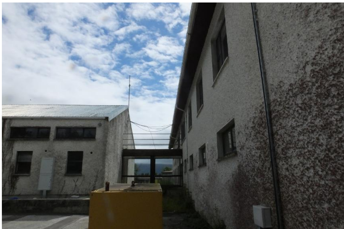
Plate 2: The corridor joining the two office buildings
