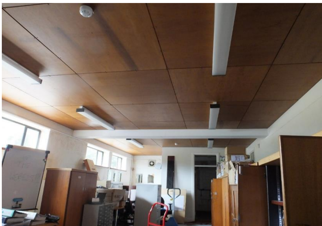
Plate 11: Offices well sealed in other areas below the main attic (1)
