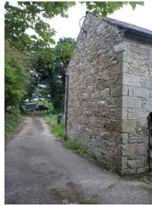
Photo E_3 - East gable/ northeast corner
