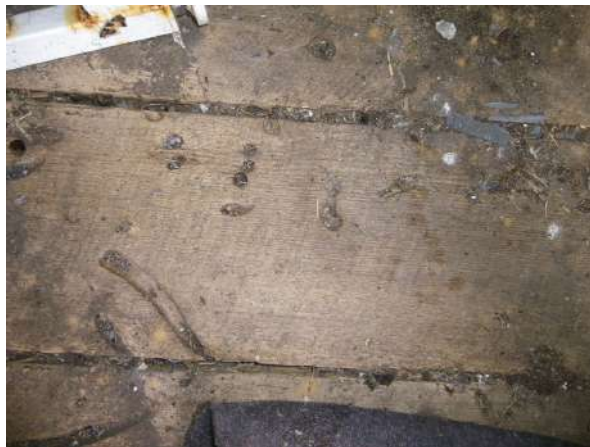
Photo F_4 Floor boards near hatch 200x20mm approx
