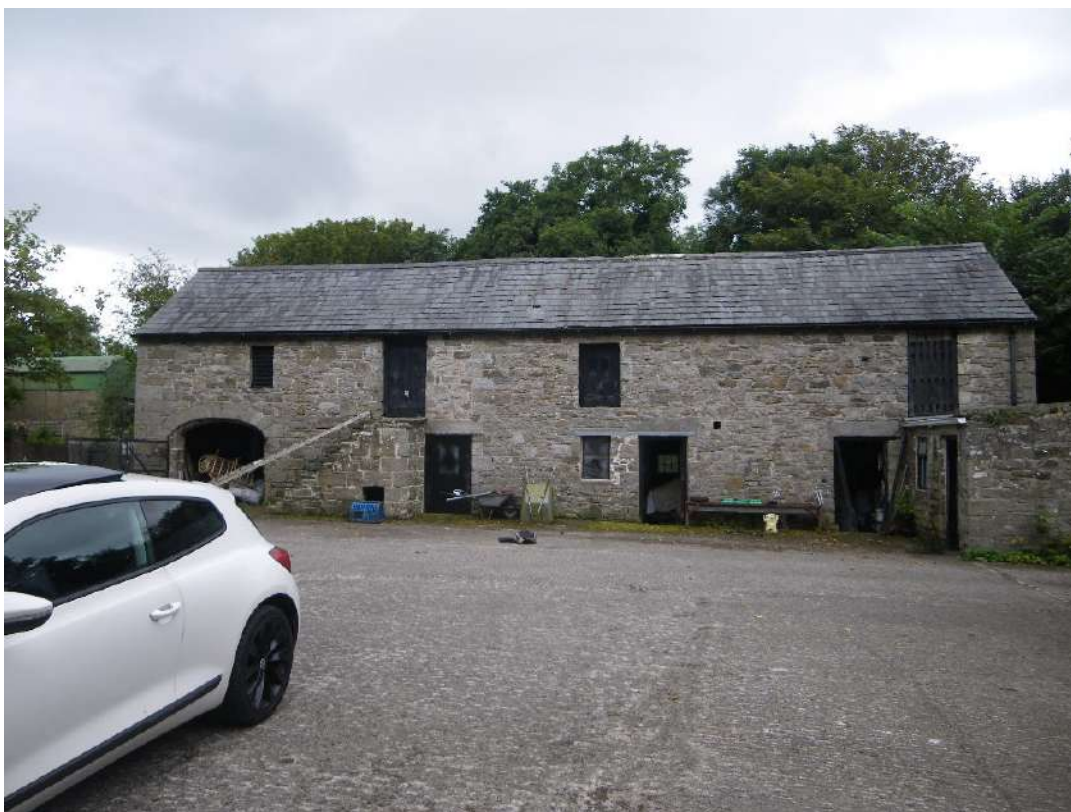
Photo E_1 - North elevation of the building
