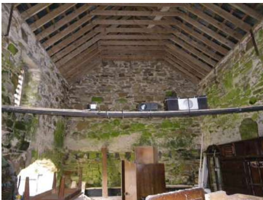
Photo C_1 Cart House looking towards east gable
