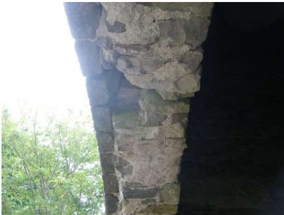
Photo A_1 Cart house arch, cut stone facing outside
