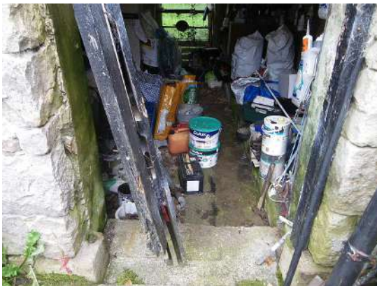
Photo D_1 Door frame to byre to be completed/ repaired
