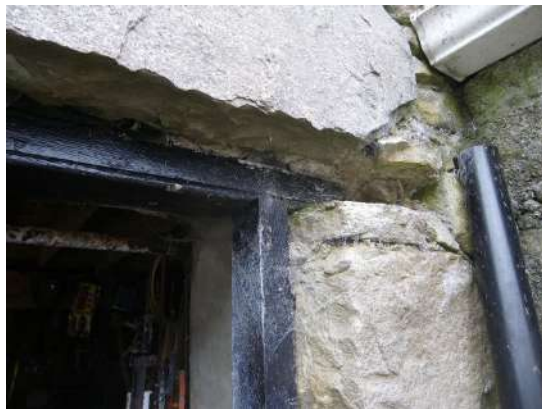
Photo D_2 Door head built into wall
