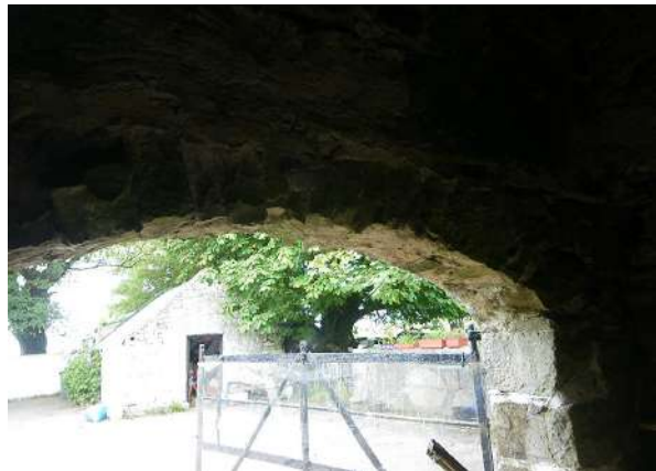
Photo A_2 Cart house arch from inside random rubble
