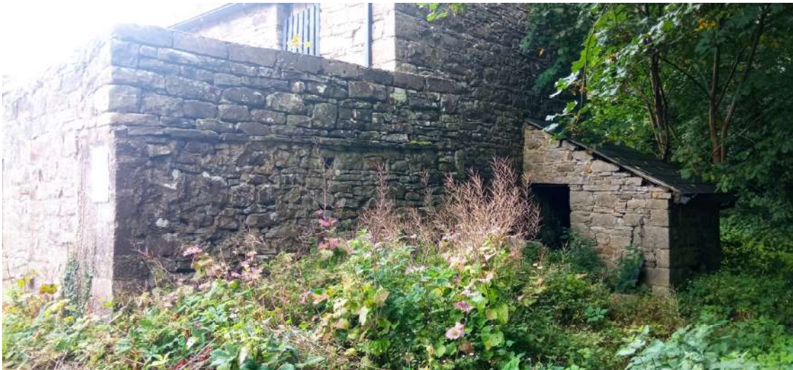
Photo E_6 North West Corner
