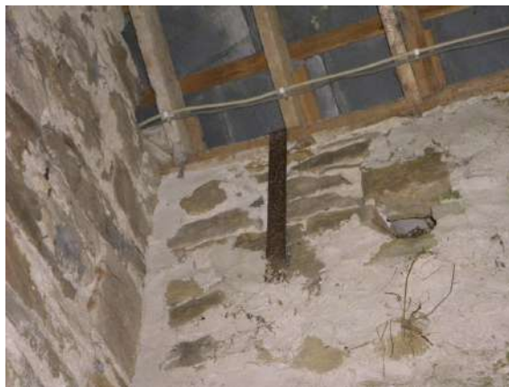
Photo C_2 Cart House wall-plate strap SE corner
