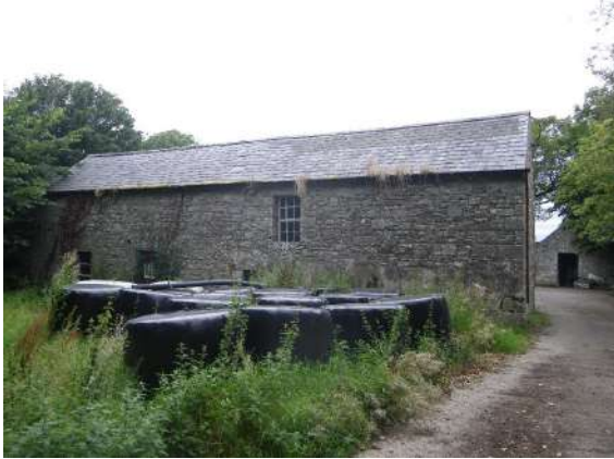
Photo E_2 South – Rear/ downpipe discharging to ground
