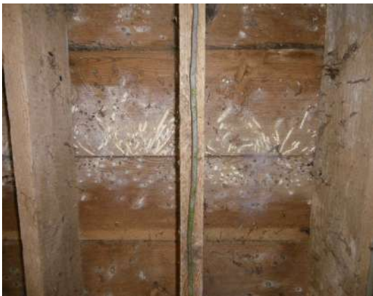
Photo F_3 Underside of floorboards in Byre
