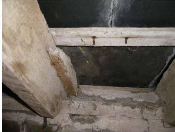
Photo R_2 Wallplate and extender/ tilting piece
