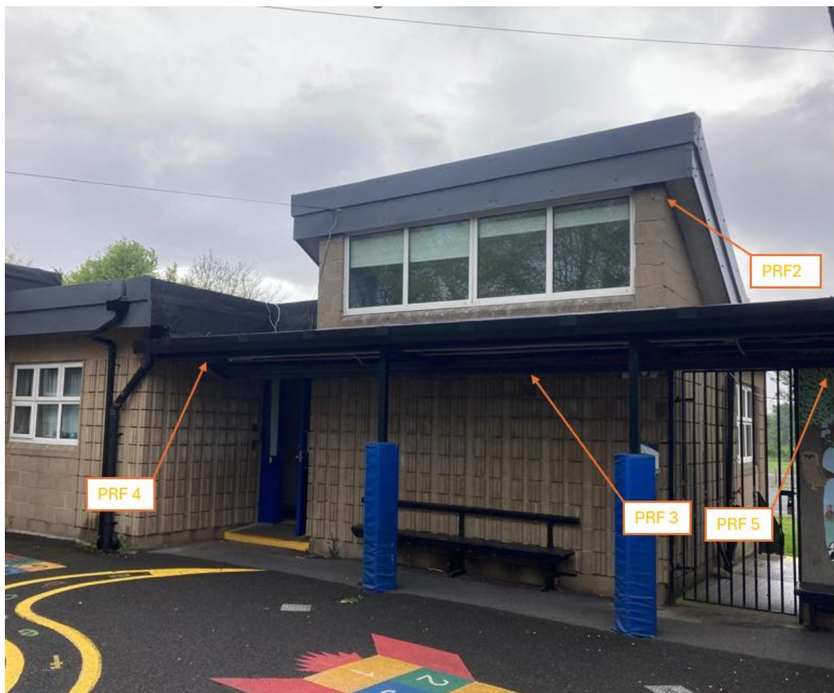
Plates 6. Previously identified (and confirmed in 2026) Entry and Exit points
