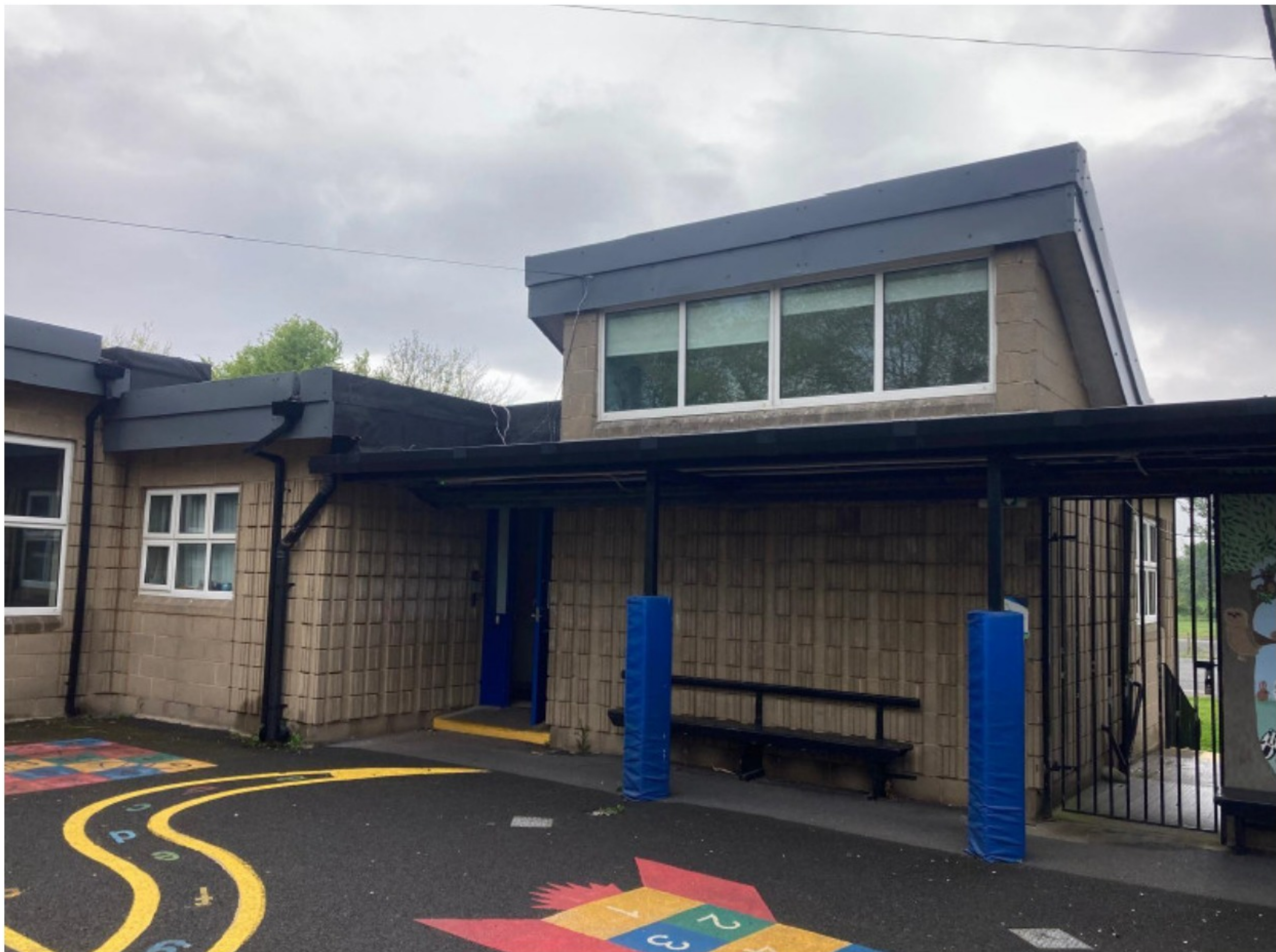
Area of existing school building where bats observed to enter/ exit the roost
