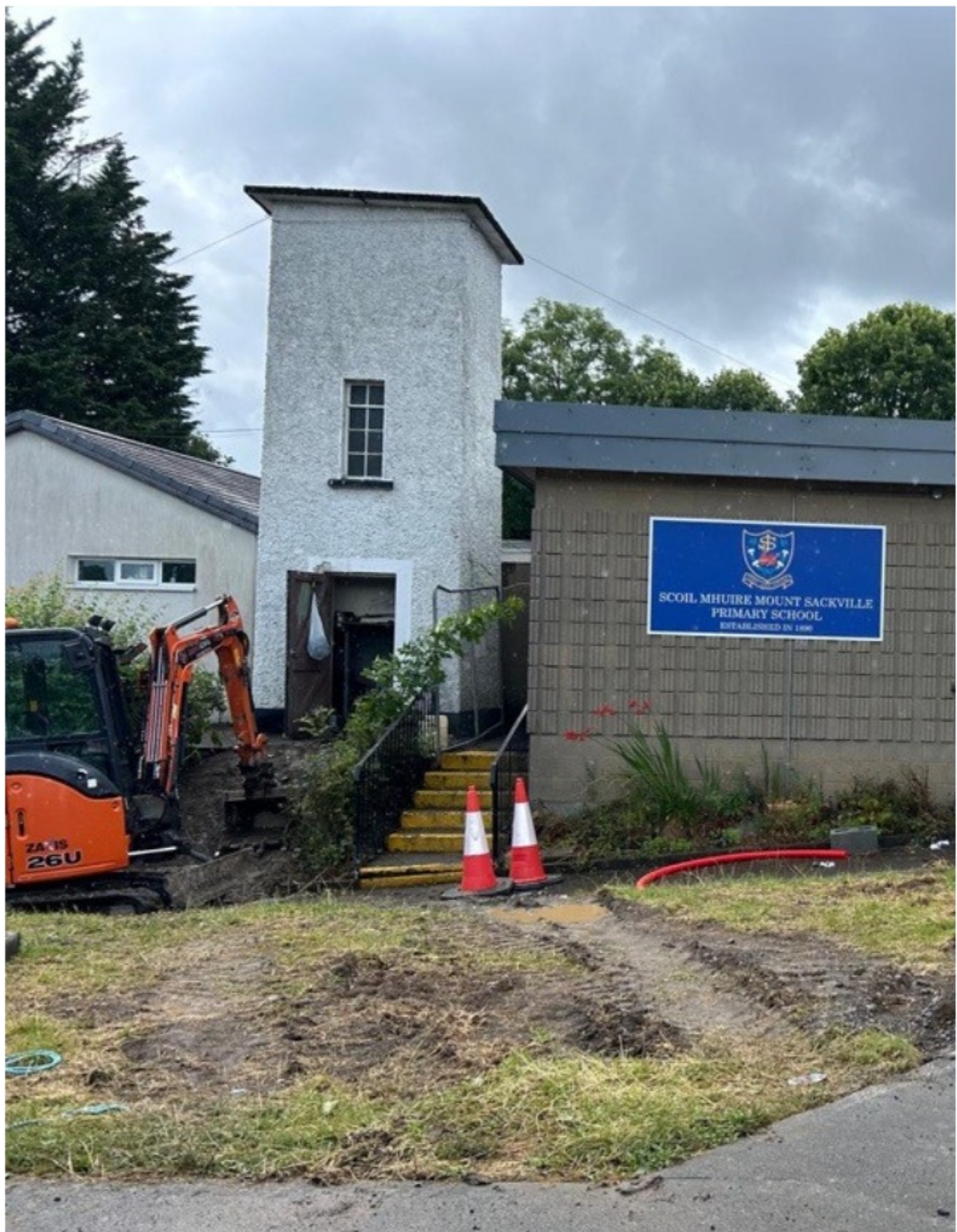
Disused Water Tower adjacent to the existing roost location within the existing school building
