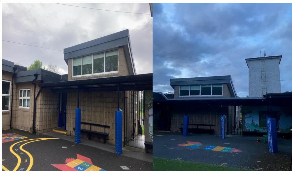
Plates 1&2 – Modular Building with Flat Roof Where Bat Roost is Located (left) and Disused Water Tower in relation to modular building (Right)
