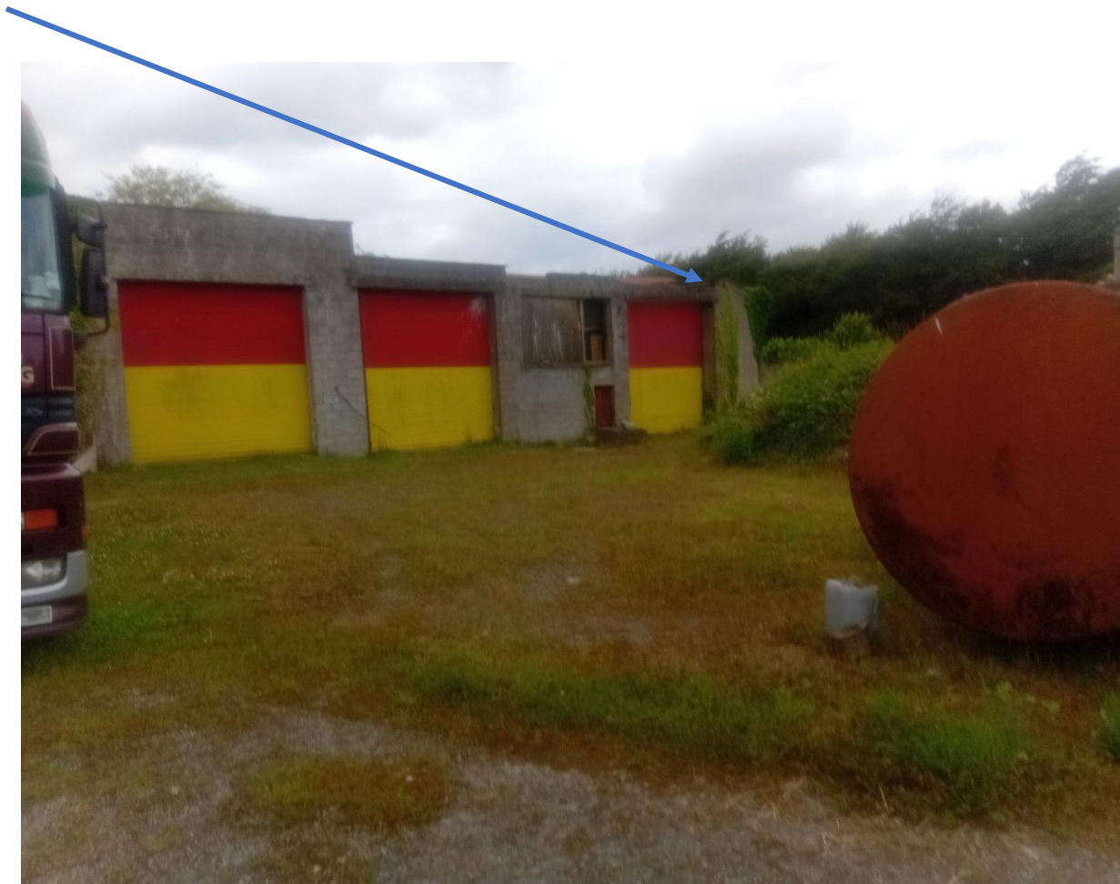
Plate 3-1 Confirmed exit point during emergent survey 2026
