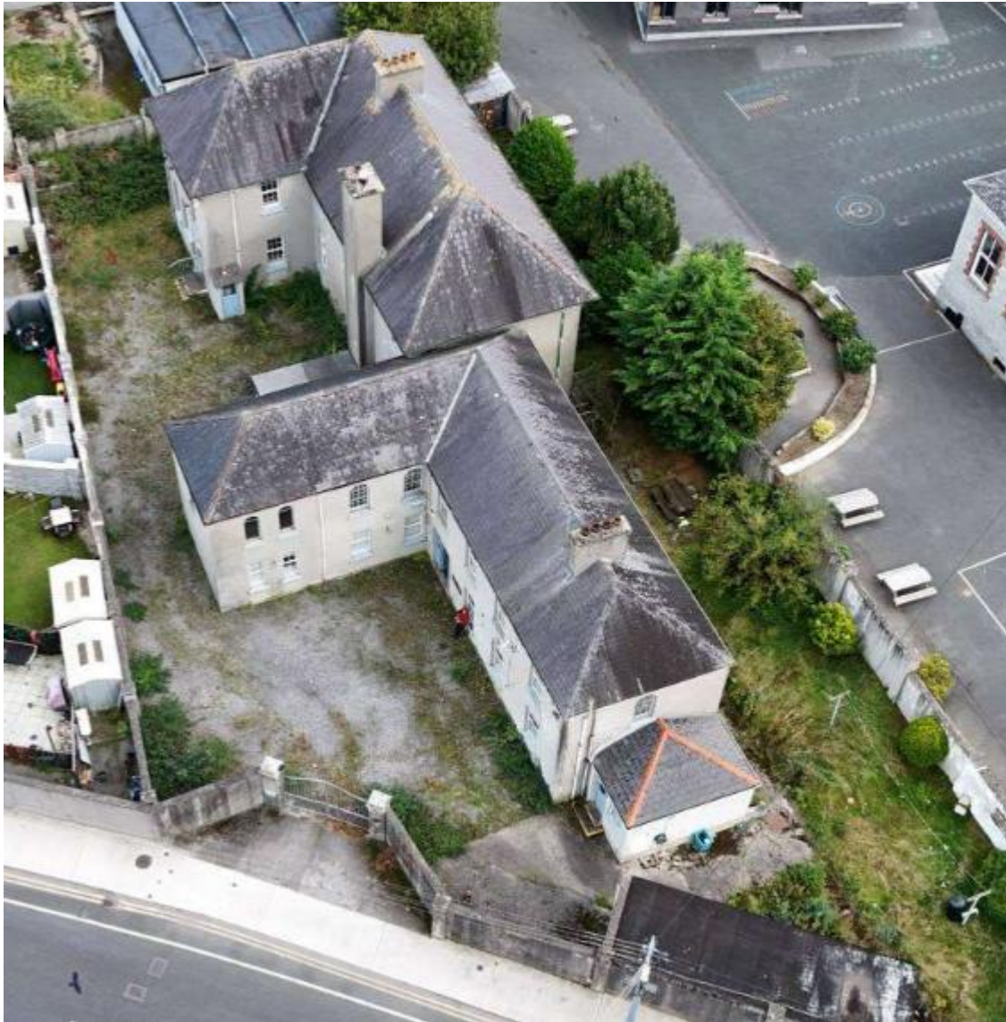
Photo of site
