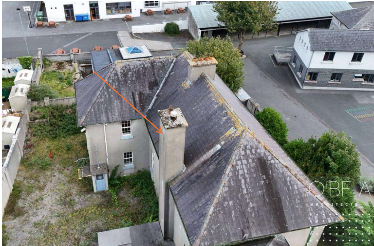
Leisler's bat roost, exit point at grille.
