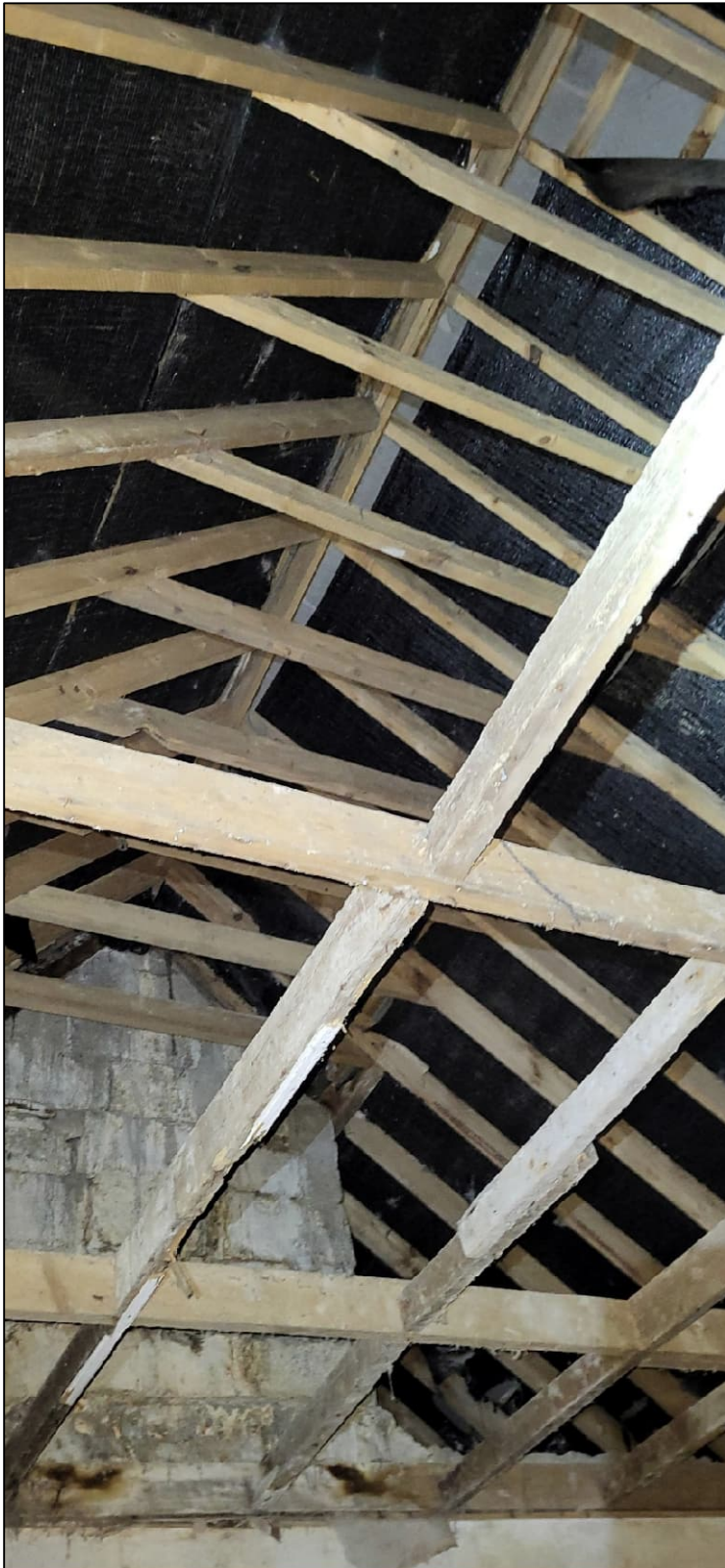
Plate 3 Open attic space and view of the inside of the roof
