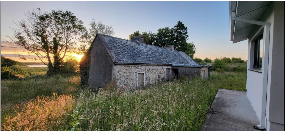
Plate 1 View from the south-east of the cottage
