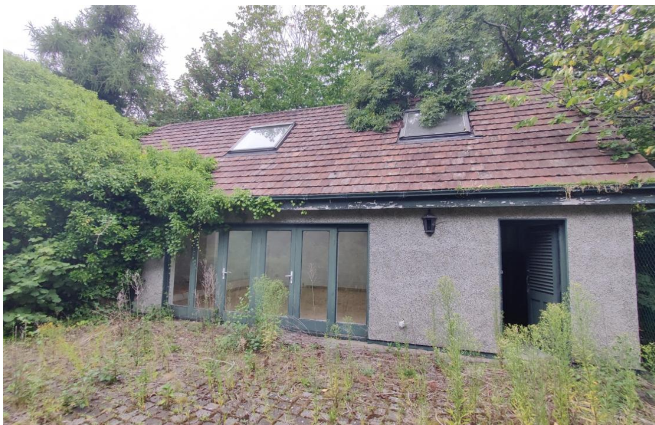
Plate 4. Small Outbuilding North of Residential Dwelling
