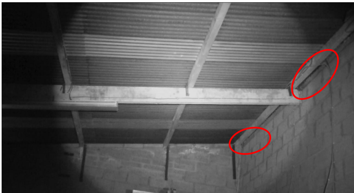
Plate 4-19: Interior of the lean-to part of the disused agricultural building; the Red circle shows crevices where bats were observed appearing from.
