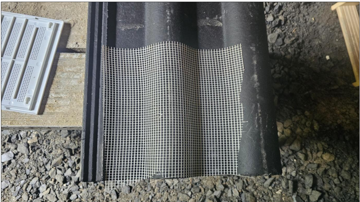
Plate 4-10. Mesh provided to ensure access to the compensatory bat roost at the roof tiles.
