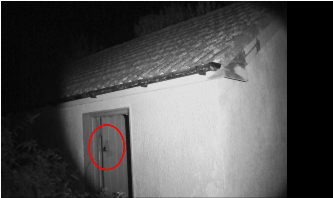
Plate 4-5: Bat access point – garage (structure 2)
