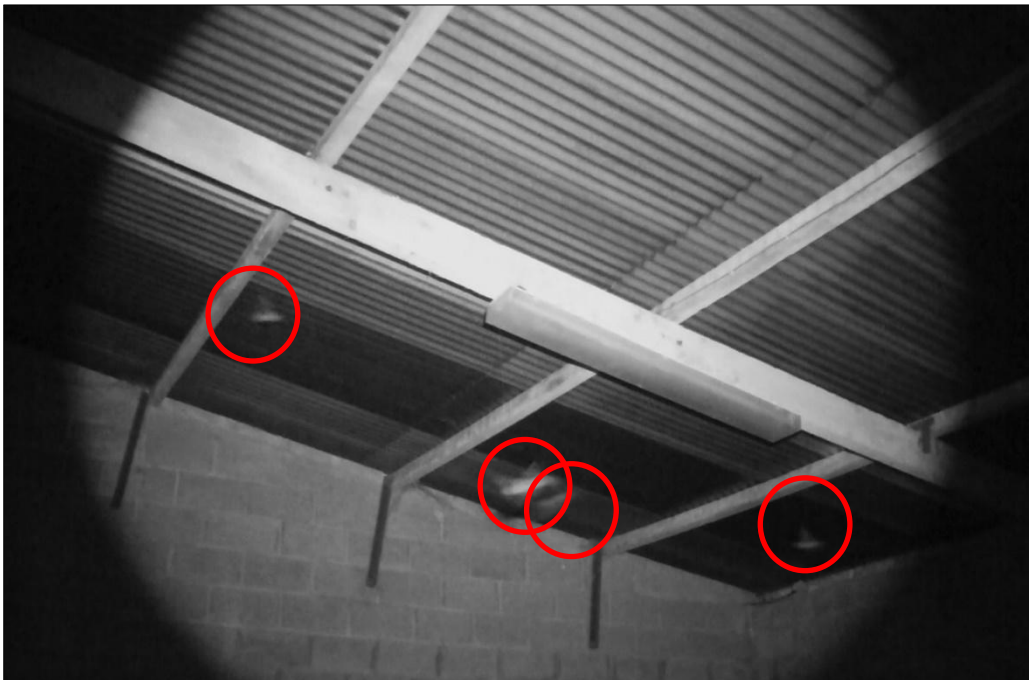
Plate 4-1: BLE flying within the lean-to portion of the disused agricultural building.
