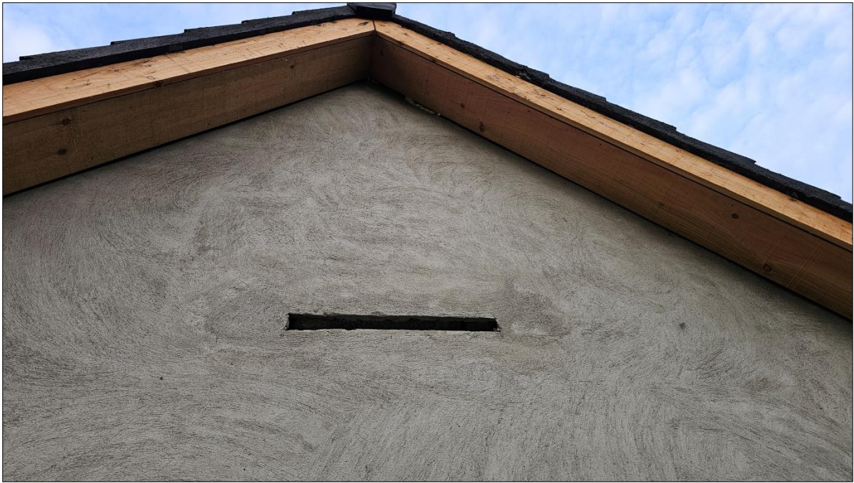
Plate 4-15. Access point to the attic space in the gable wall.
