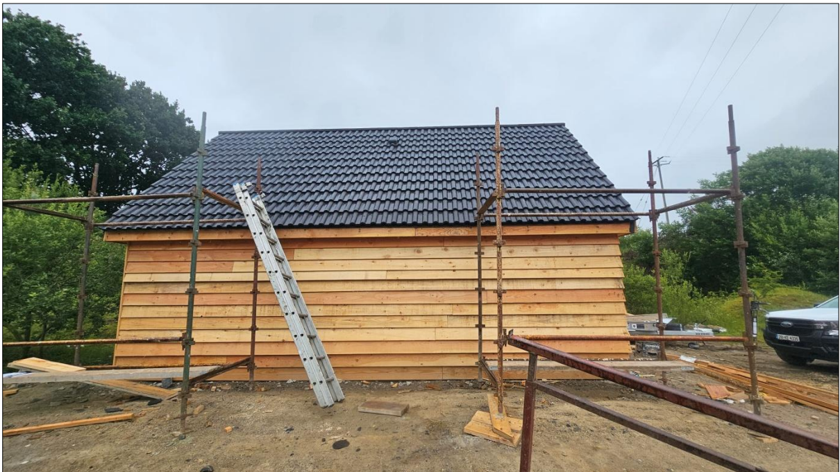
Plate 4-8. Compensatory bat roost under construction.
