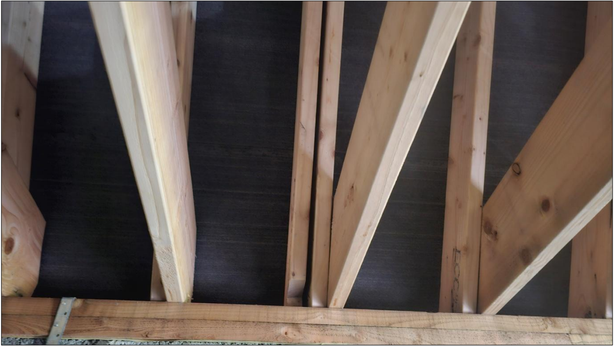
Plate 4-11. Doubling up of roof timbers to provide crevices within the attic of the bat roost.
