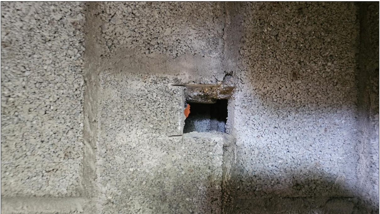
Plate 4-12. Access points to crevices within the block walls of the bat roost – providing potential hibernation sites.
