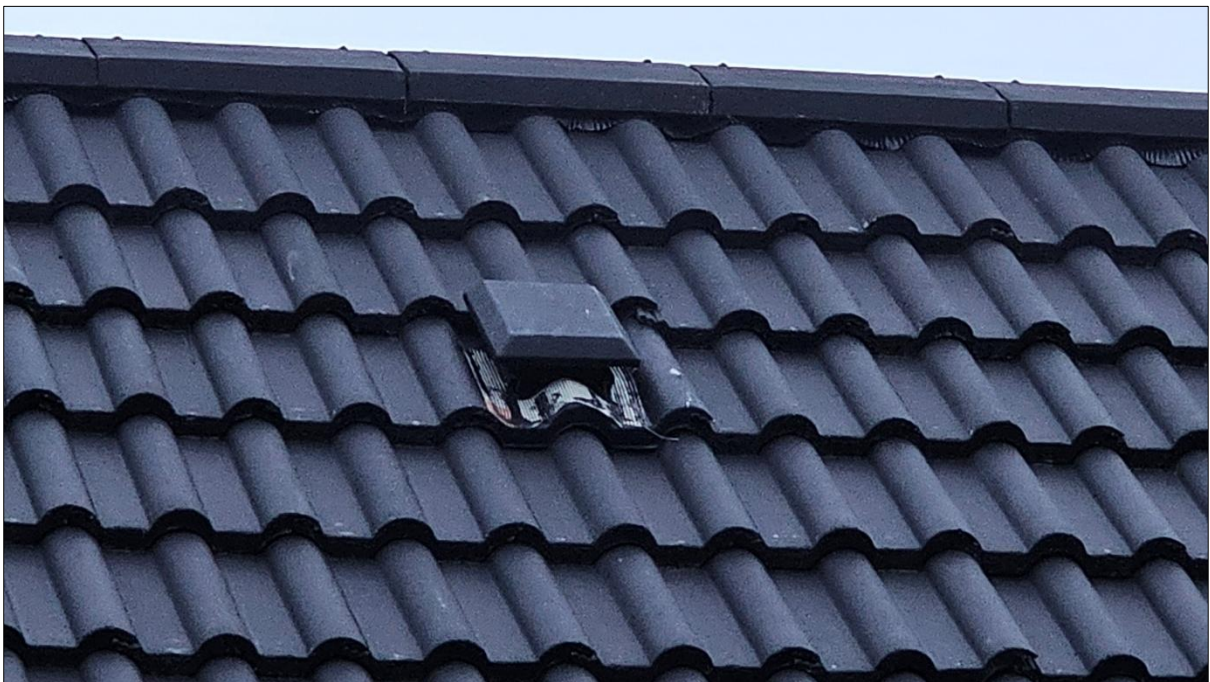
Plate 4-16. Mesh on the access point to the attic space from the roof tiles.
