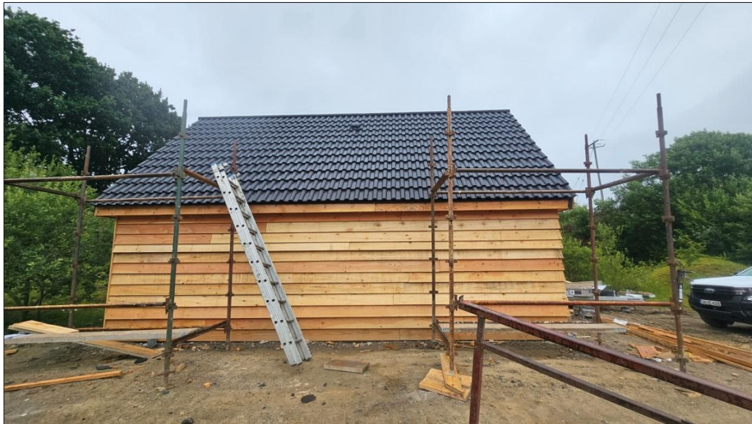
Plate 3. Compensatory bat roost under construction.
