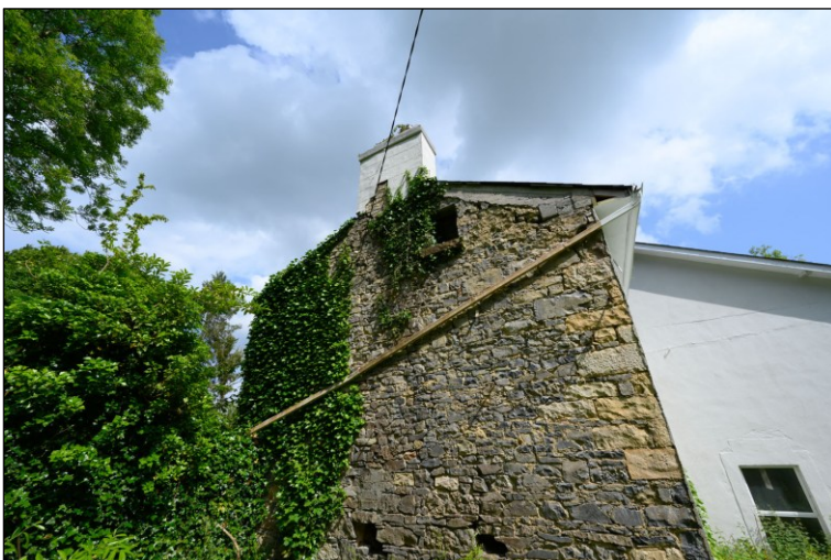
Plate 3 Rear of the house – bats are roosting in this area.
