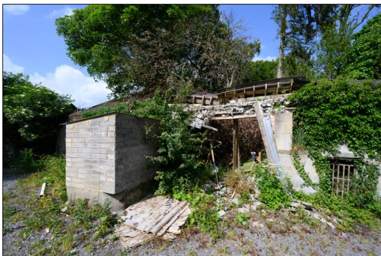
Plate 5 Outbuilding on the north side of the main house.
