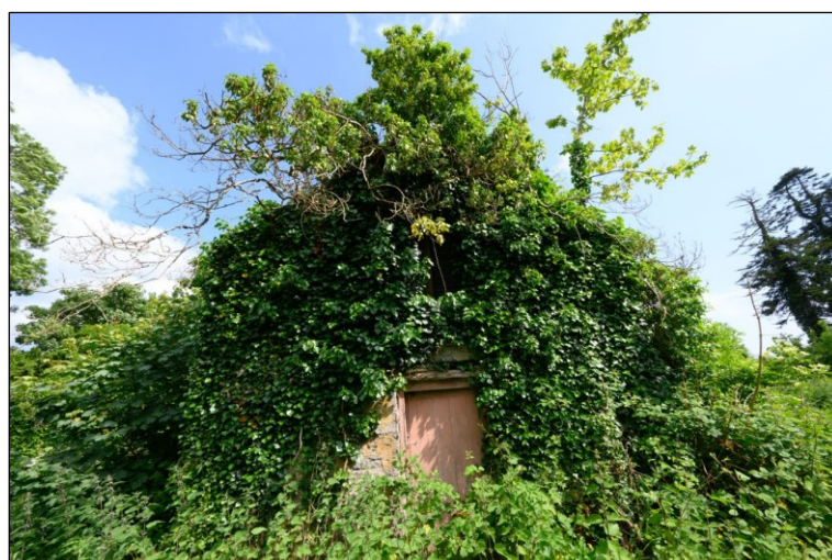
Plate 9 Building on the site that has bat potential (not directly affected, not surveyed).
