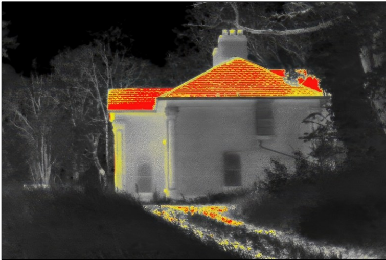
Plate 1 The subject house (thermal image).
