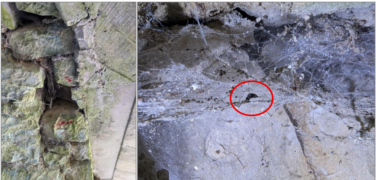
Plate 3. An additional roosting stone crevice toward the NE side of the bridge (left photograph) where bat roosting of Natterer's Bat was confirmed by DNA analysis of a single dropping that was caught in spider webs, circled in red
