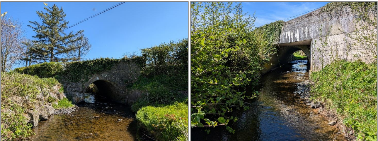
Plate 1. Views of Skerry Bridge, L2095 road, Mountmellick from the south-west (left) and north-east (right)
